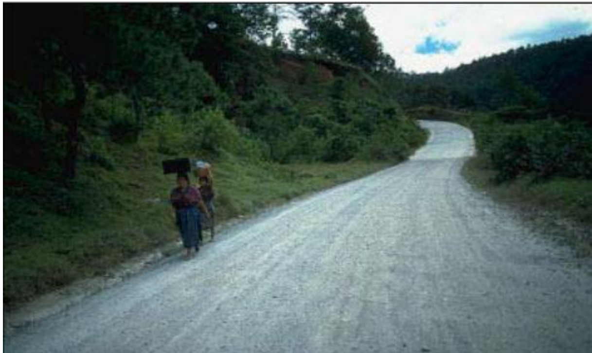
Figure 2- 1 The project site road
