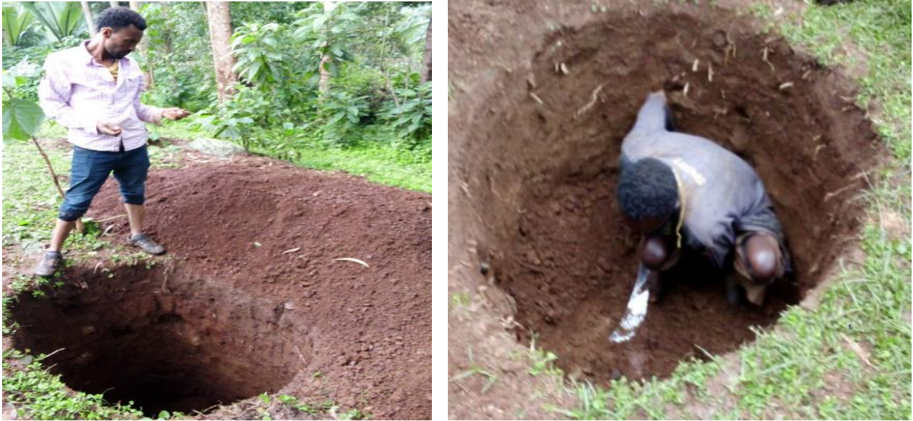
Figure 3-3: Open pit for taking sample soil test (15/10/2013)
