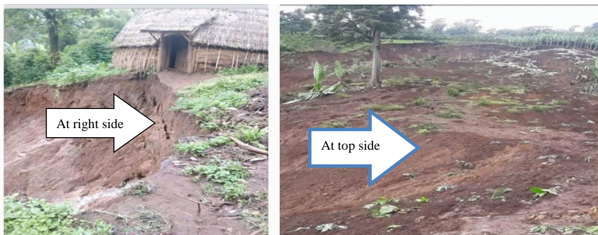
Figure 4-13: Surface damage due to landslide of Tulu Gola landslide
