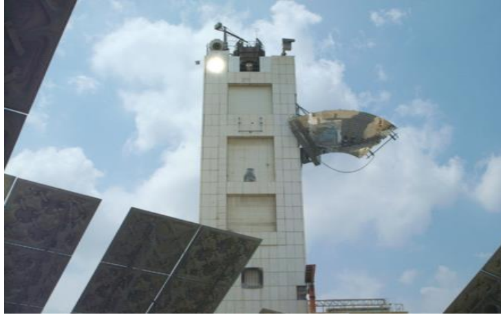
Figure 2.2: Beam down the solar field at Weizmann Institute of Science [23].
