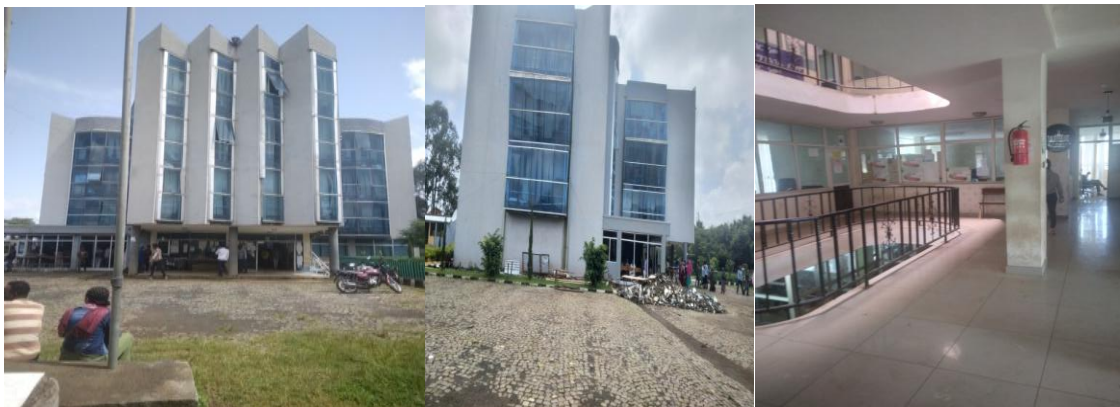
Figure 4.4: Town Administrative Building fire extinguisher equipment backyard parking space (source by author, 2023)
