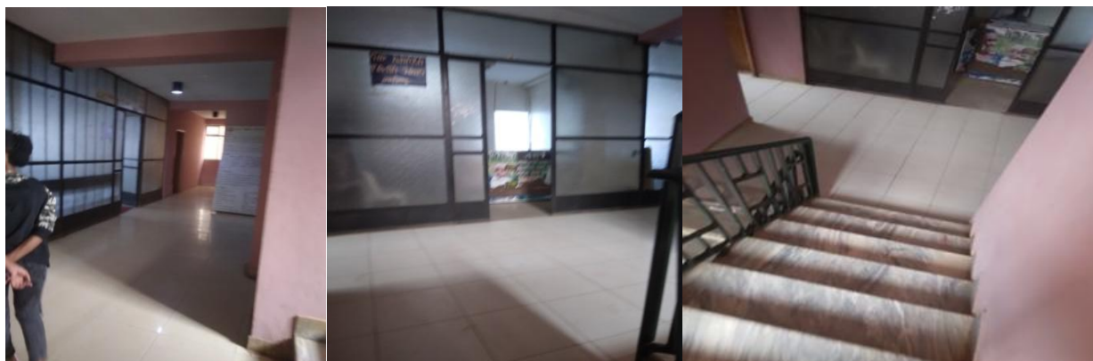
Figure 4.15. Teka Building natural lighting and ventilation (Source by Author, 2023)
