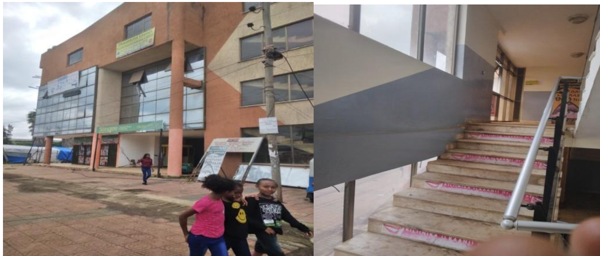
Figure 4.19. Post office building source (Source by authors, 2023)
