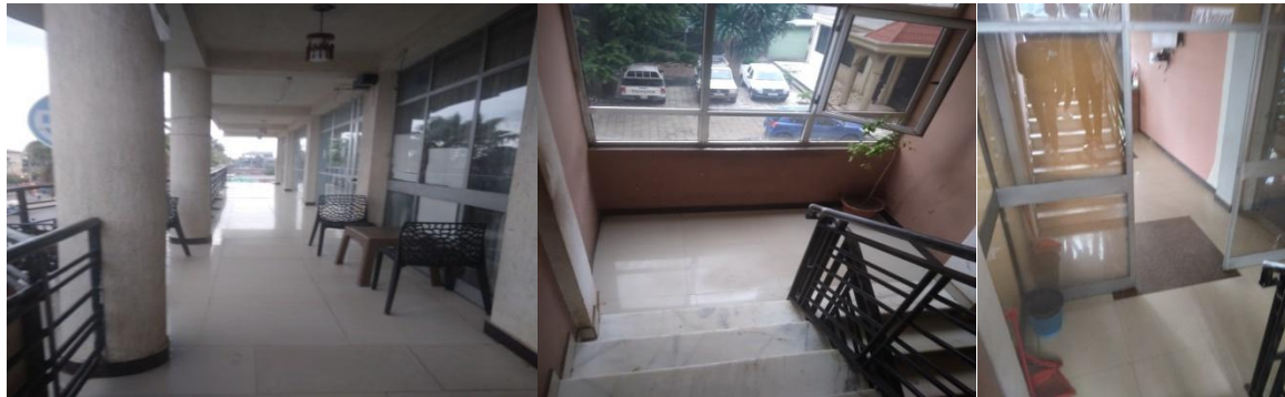
Figure 4.9. Haro Wonchi Building natural lighting and ventilation (Source by Author, 2023)
