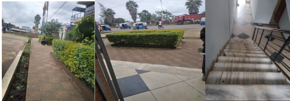
Figure 4.23. Open spaces around post office building (Source by Author, 2023)
