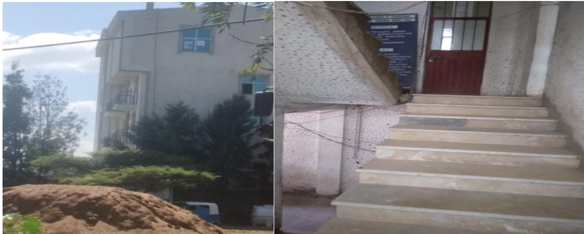
Figure 4.29. Open spaces around post office building (Source by Author, 2023)
