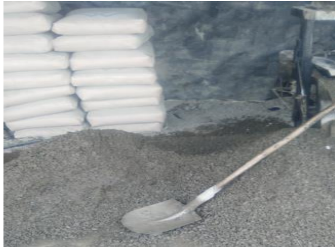
Figure 4.2 Storage of cement near concrete mixing area
