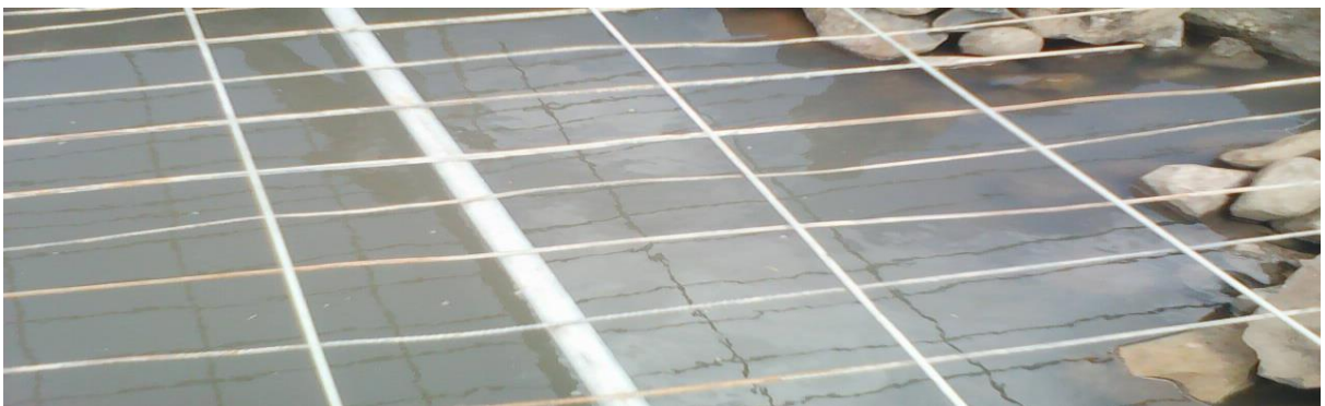
Figure 4. 11 partially covered spring box during construction
