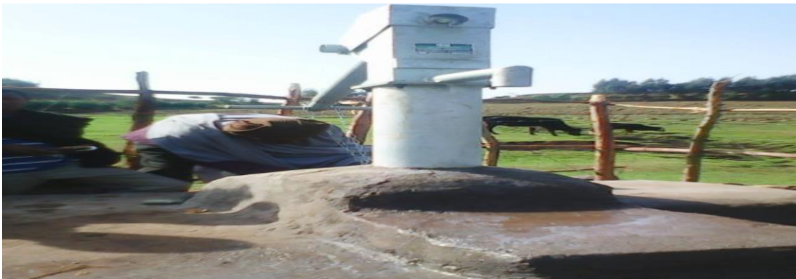
Figure 4. 16 A hand dug well after construction
