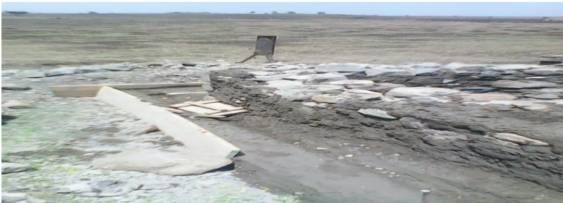
Figure 4. 15 A hand dug well during construction
