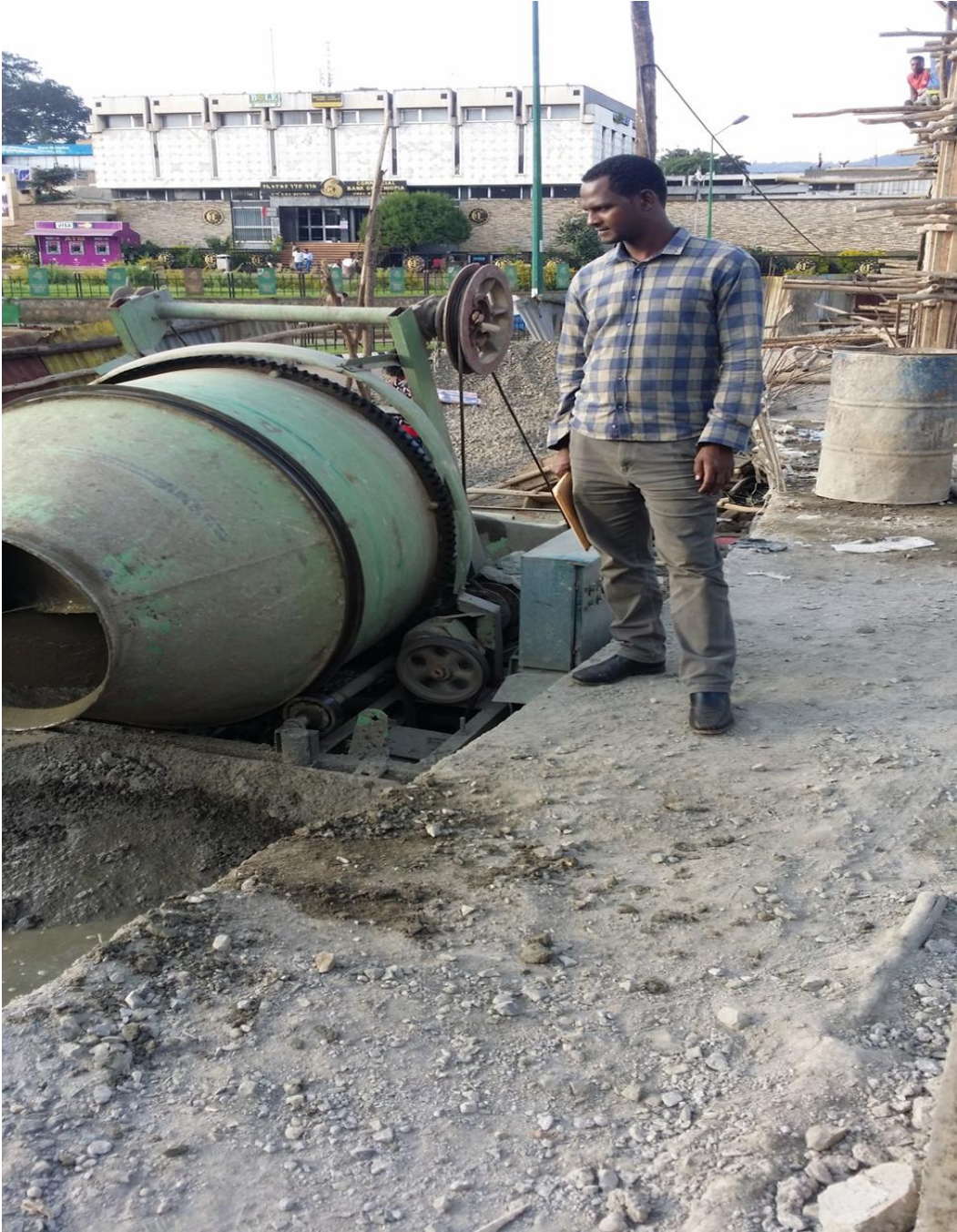
Figure 10 350liter Stationary concrete mixer used
