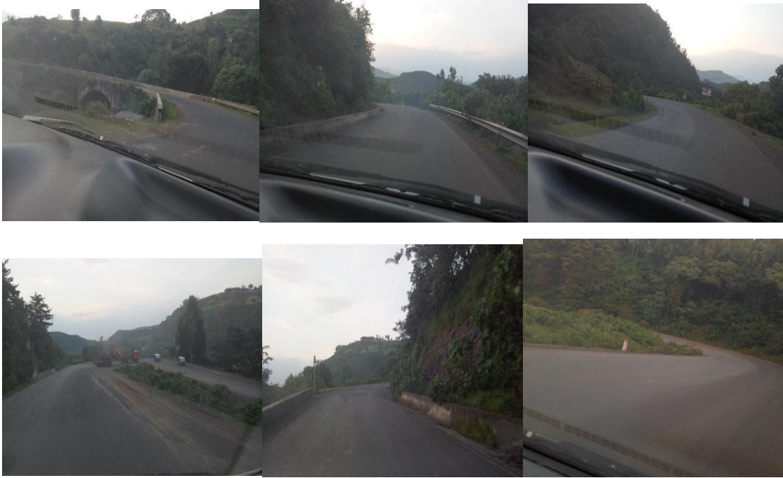
Figure: curves with insufficient sight distance, steep slope and sharp curves
