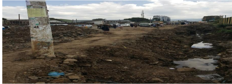
Figure 4.12: Mexico – Amestegna road project
