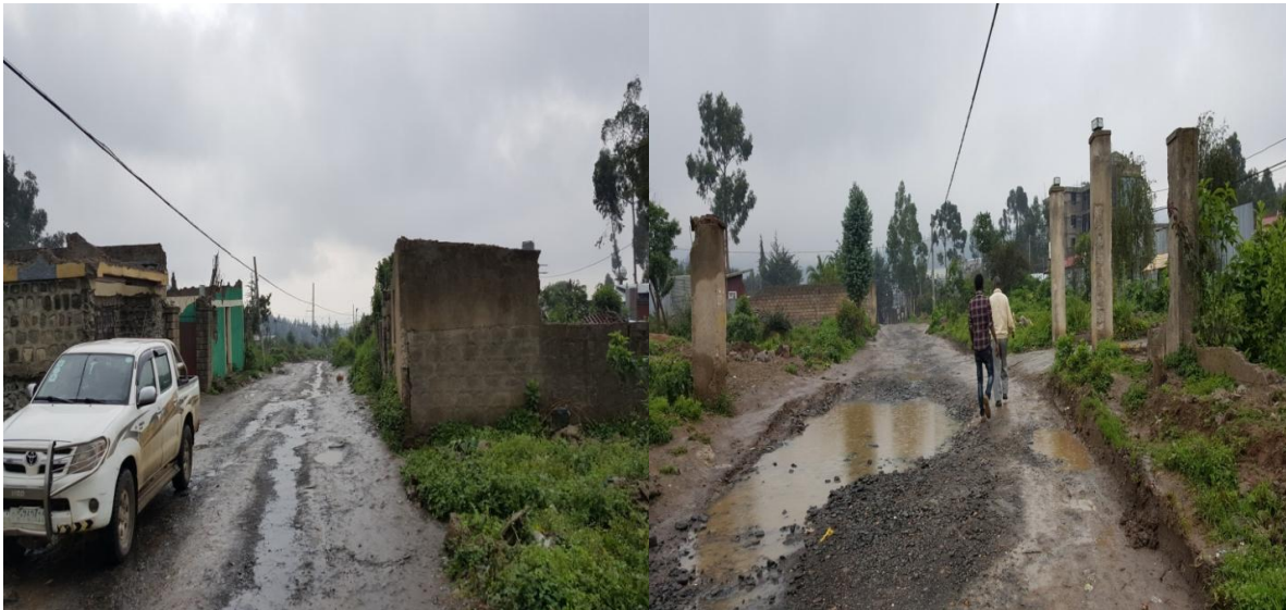
Figure 4.4: CMC Roundabout – Karalo Junction Asphalt Concrete Road Construction
