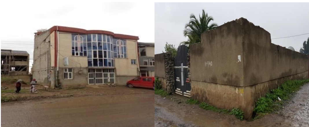
Figure 4.22: Affected existing houseson Betel-alembank and Cmckaralo junction
