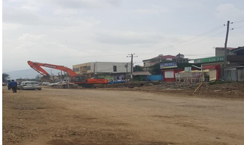
Figure 4.15: The Construction Works for B/Gebriel- Abo roundabout asphalt road project.
