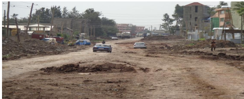
Figure 4.13: Kadisco paint factory to crown hotel road project
