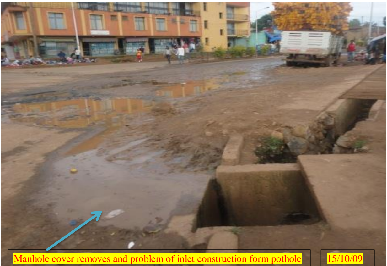
figure 4.12 assessment of drainage construction
