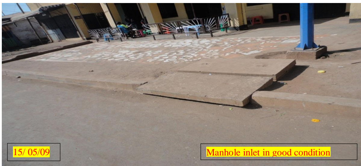
figure 4.4 manhole inlet in good condtion
