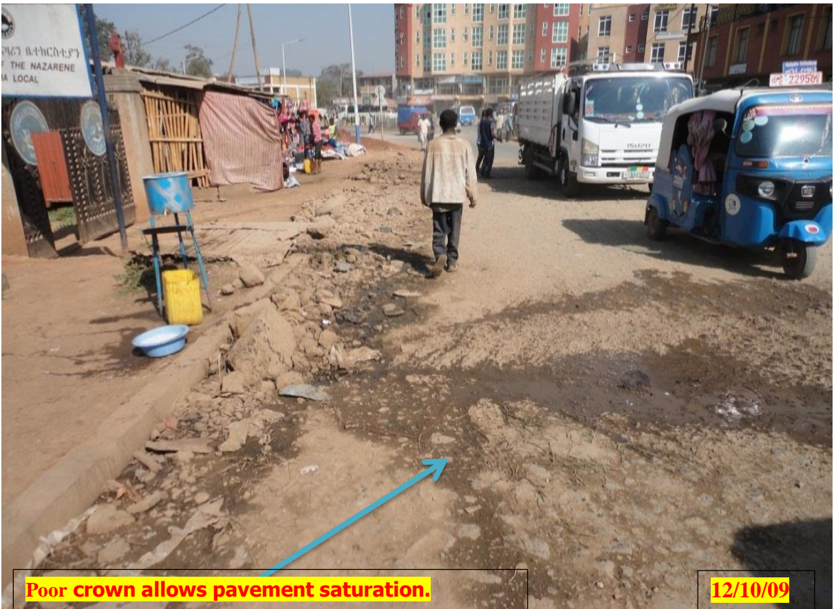
Figure 4.20 shows that pavement failure and inlets doesn't work (in front of genu hotel)
