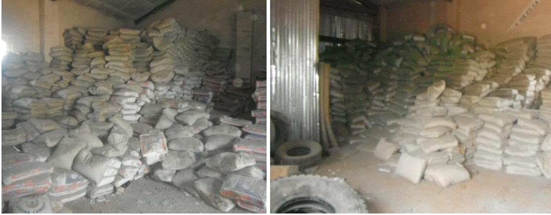
Figure 4.2 Storage of cement on the construction sites (varnero site)
