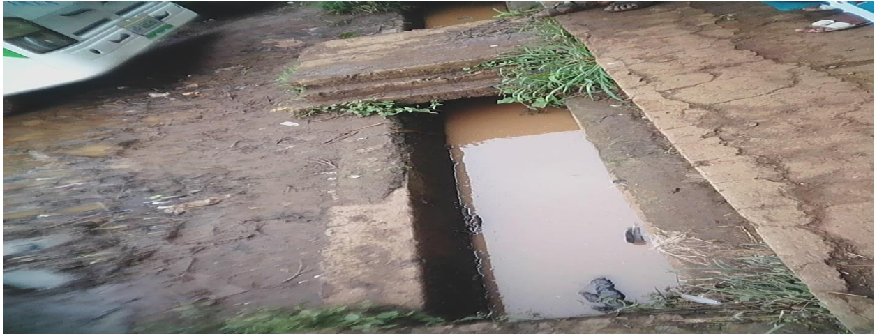
Figure 4.13: Picture indicating sewerage of terminal (taken by researcher).
