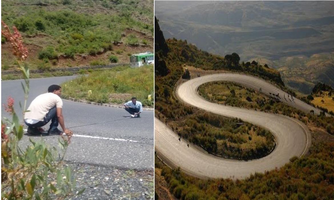
Figure 3.9: Field measurement photos taken at No. five road section.
