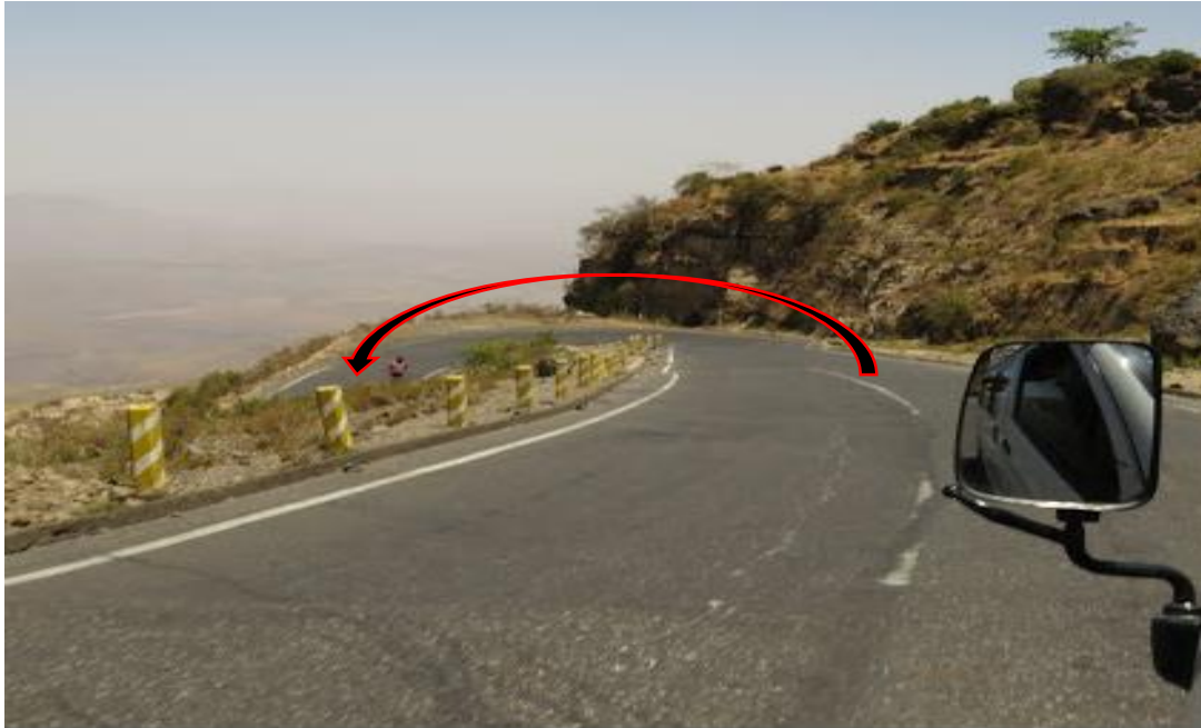
Figure 3.10: Field photo with a sharp horizontal curve and difficult downgrade at Gelgele section.
