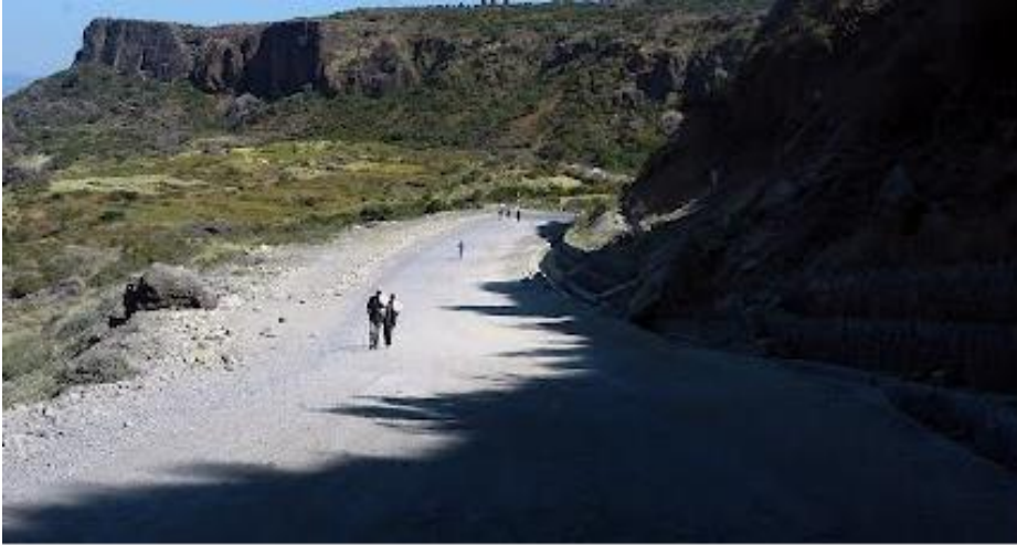
Figure 3.11: Field measurement photo with bad wearing surface at Dembeza Road section.
