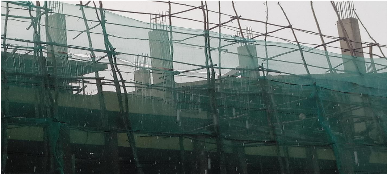
Figure-4.12: Building construction in Jimma
