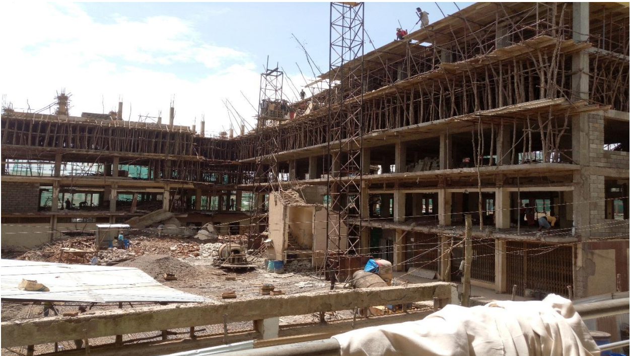
Figure-4.11: Demolishing and construction site in Jimma
