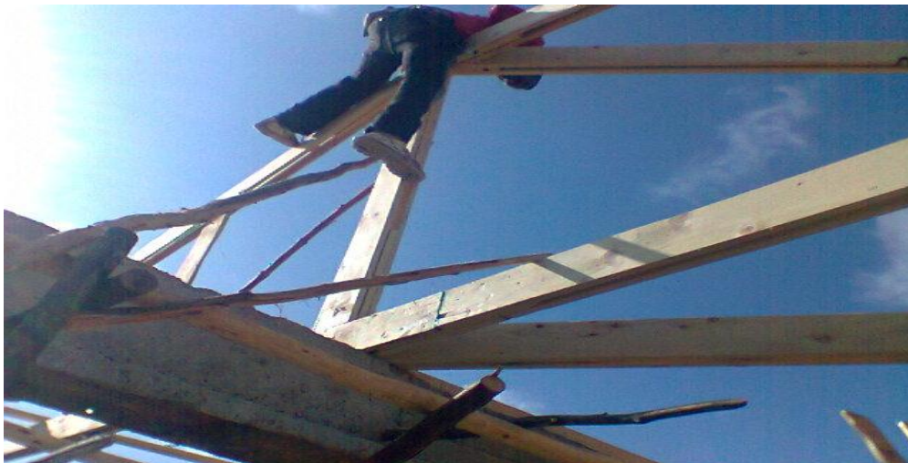
Figure- 4.13: Building construction in Jimma
