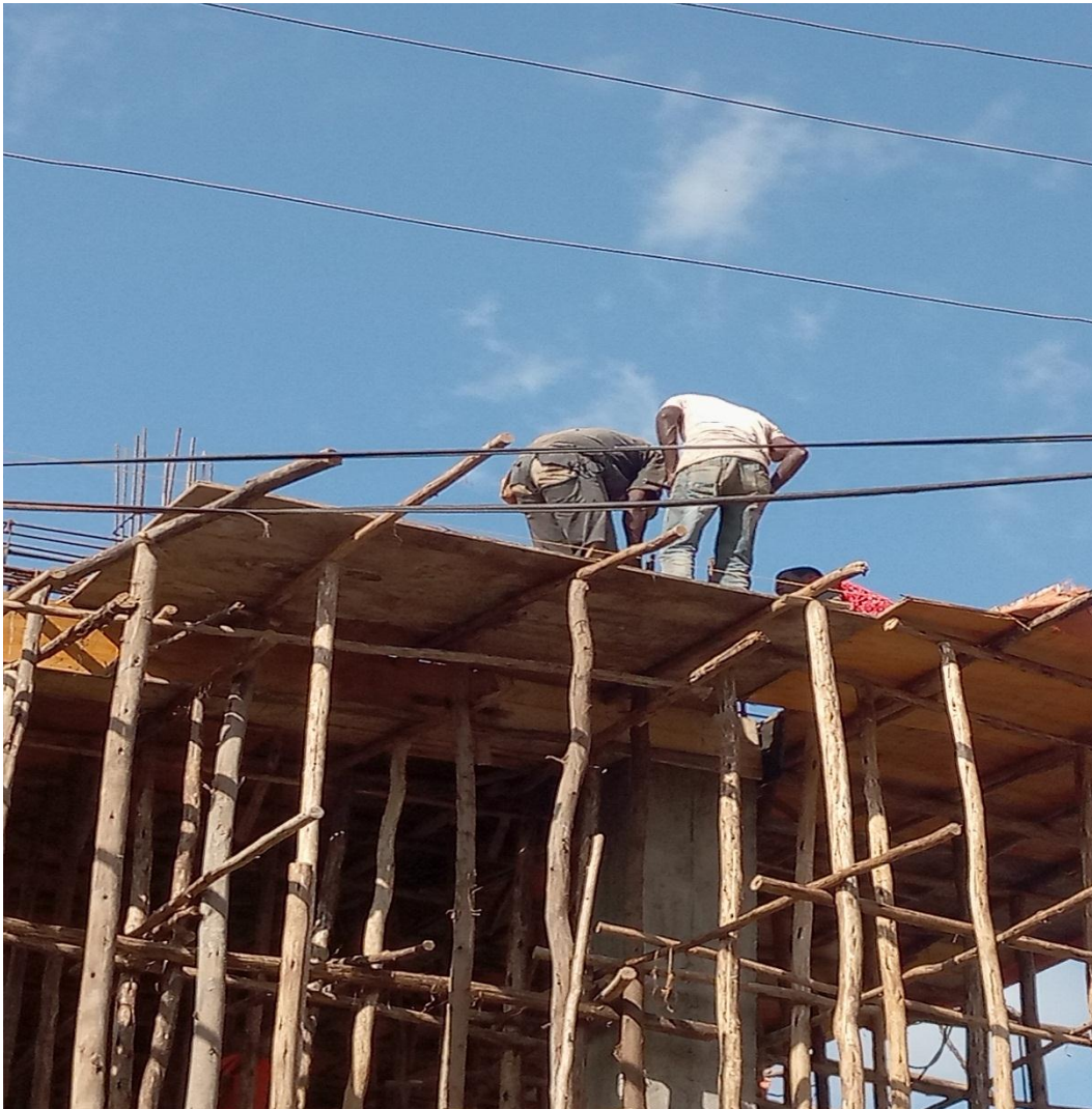
Figure -4.8: Building construction in Jimma
