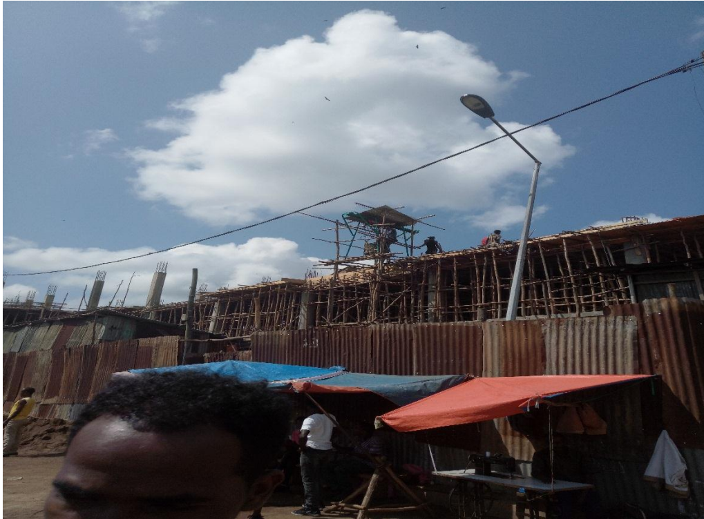
Figure-4.9: Building construction in Jimma
