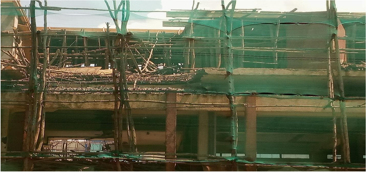
Figure-4.10: Demolishing and construction site in Jimma
