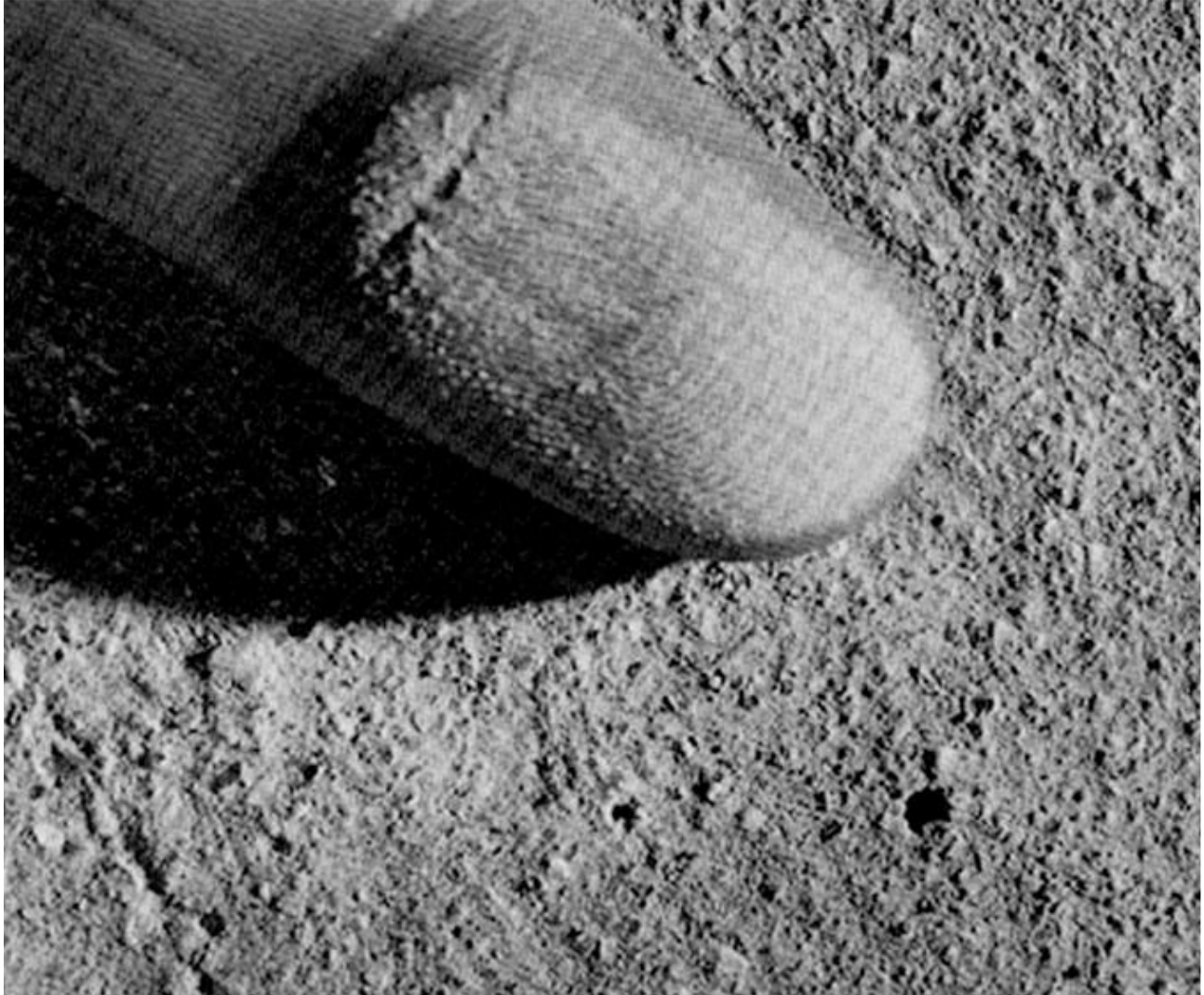
Figure 5 Dusting evident by the fine powder that can be easily rubbed off the surface
