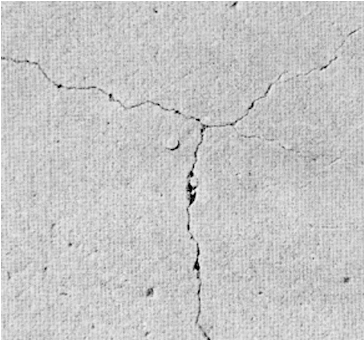
Figure 2 Drying-shrinkage cracks
