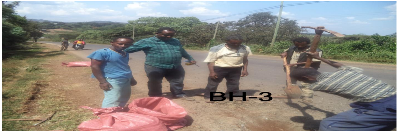
Figure 3.3 Borehole BH-3 at station 386+000 (30-Nov-15)
