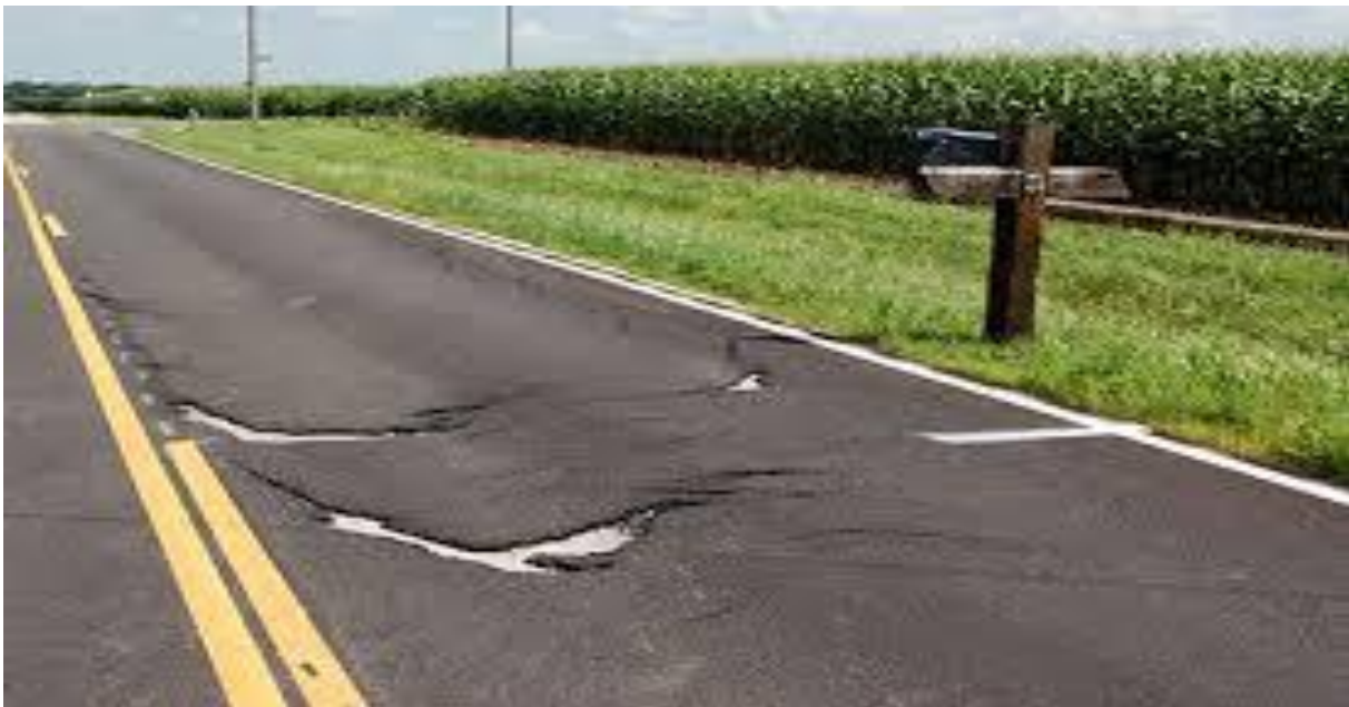
Figure 2.16: Delamination of an overlay (Miller, J. S., Rogers, R. B. and Rada, G. R., 1993)
