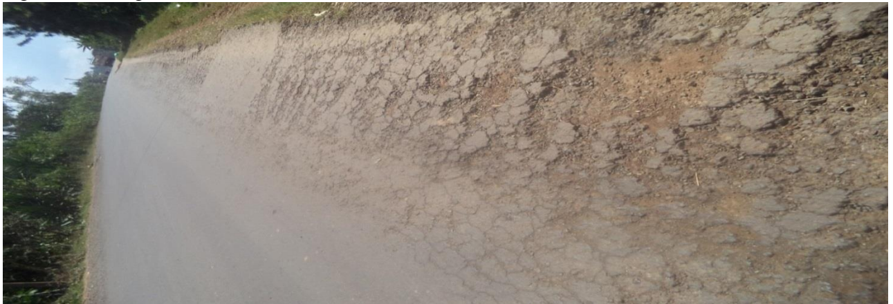
Figure 4.2: Alligator cracks (29-Nov-15)
