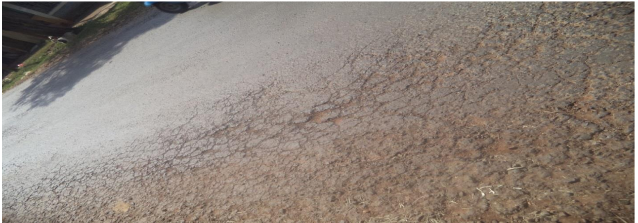
Figure 4.2: Alligator cracks (29-Nov-15)
