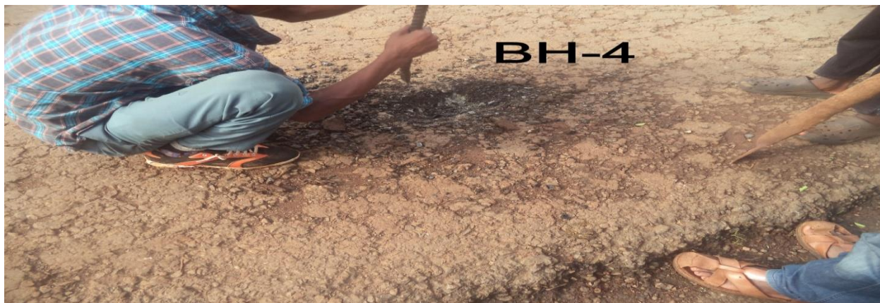
Figure 3.4 Borehole BH-4 at station 397+000 (30-Nov-15)
