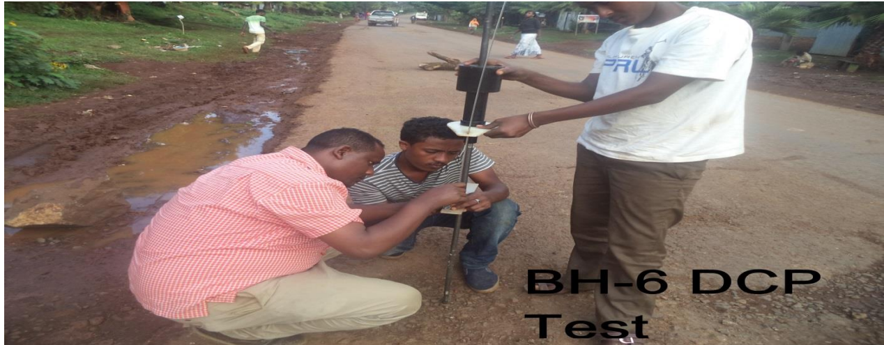
Figure 3.6: Borehole Number BH-6 (Lat7°51'12.5568'N & Lon. 36°35'46.1859'E) DCP test (9 December 2015)
