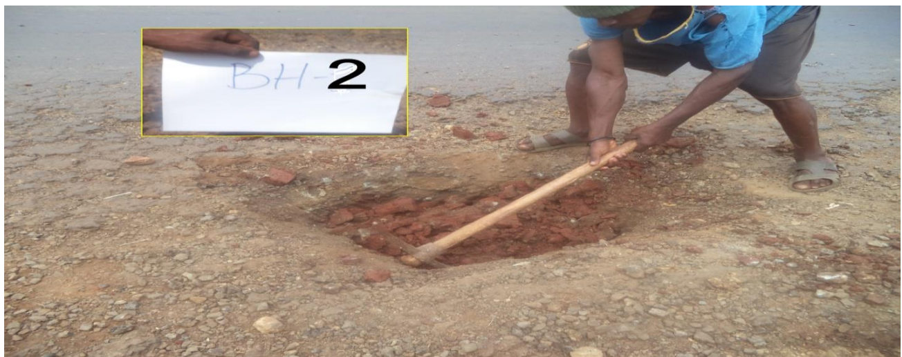
Figure 3.2 Borehole (BH-2) at station 398+000 (29-Nov-15)
