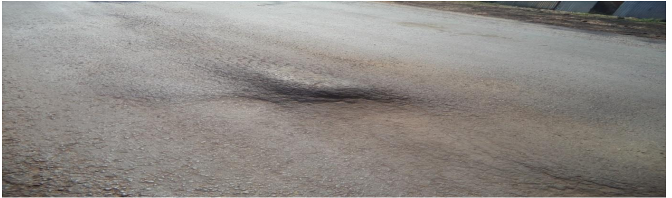
Figure 4.1: Shoving or Corrugations (29-Nov-15)
