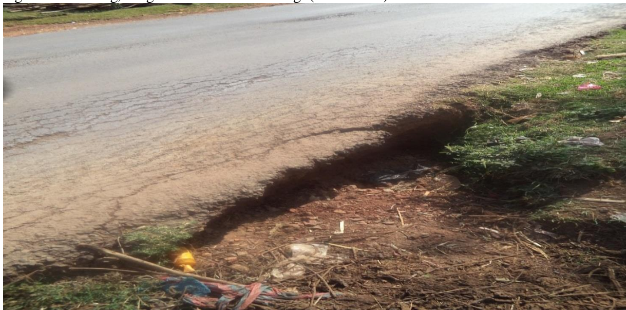
Figure 4.7: Rutting, alligator cracks and shoving (29-Nov-15)
