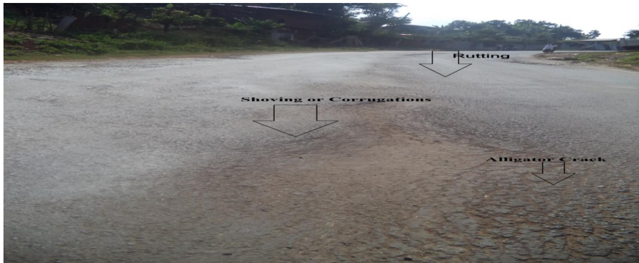
Figure 4.7: Rutting, alligator cracks and shoving (29-Nov-15)
