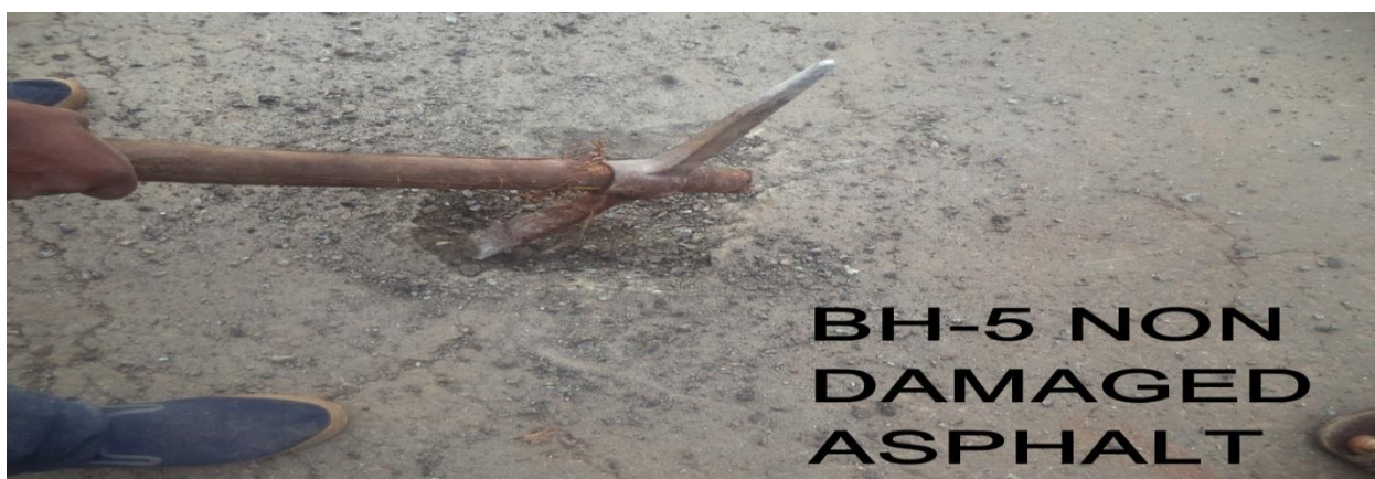
Figure 3.5 Borehole BH-5 at station 396+000 none damaged Asphalt for comparisons. (30-Nov-15)
