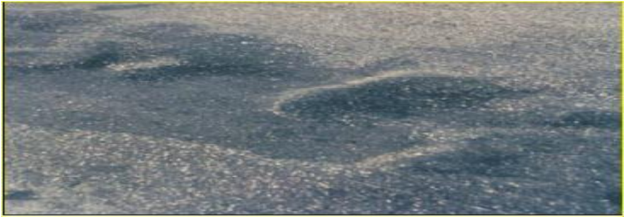
Figure 2.9.Corrugation and Shoving. (Miller, J. S., Rogers, R. B. and Rada, G. R., 1993)
