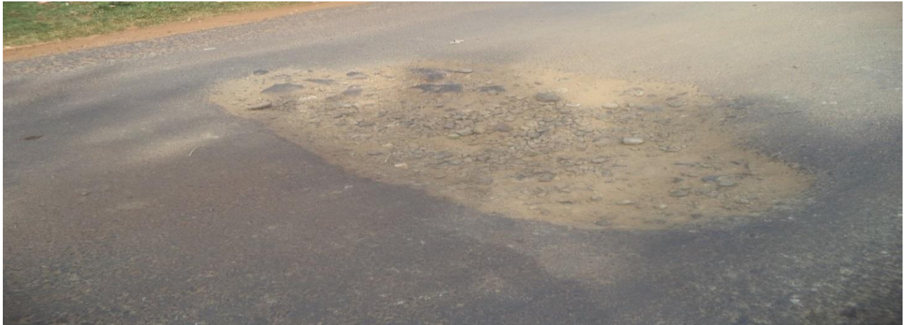
Figure 4.4: Potholes (29-Nov-15)
