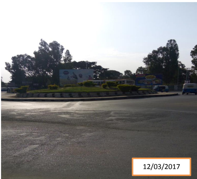
Figure 4.3 Feature of roundabout below Awasho bus station
