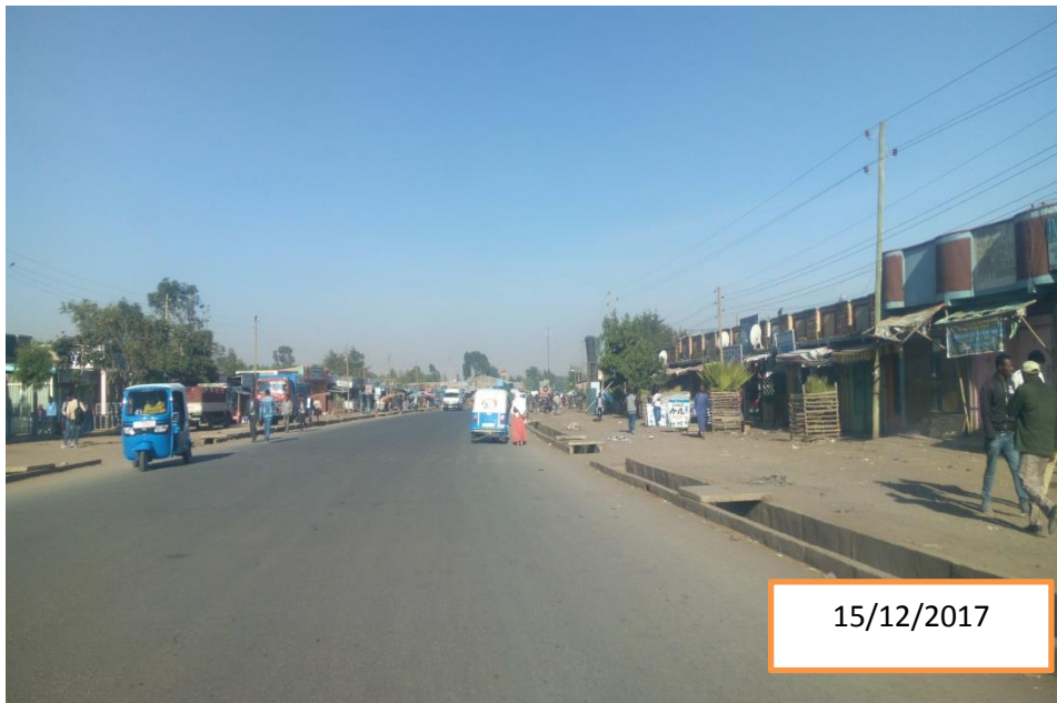
Figure 4.10 Adaba town road section
