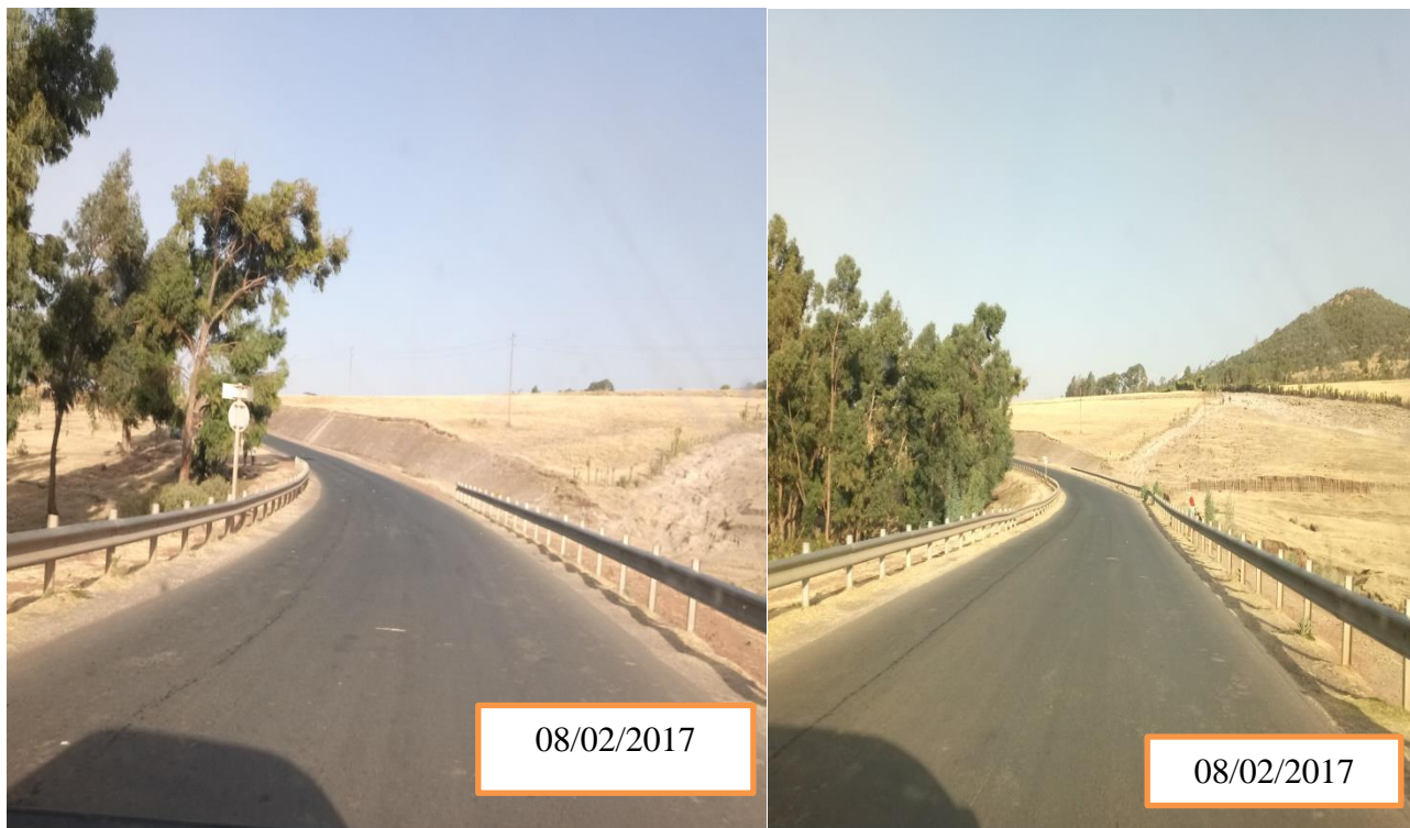
Figure 4.9 Kora Bridge sections
