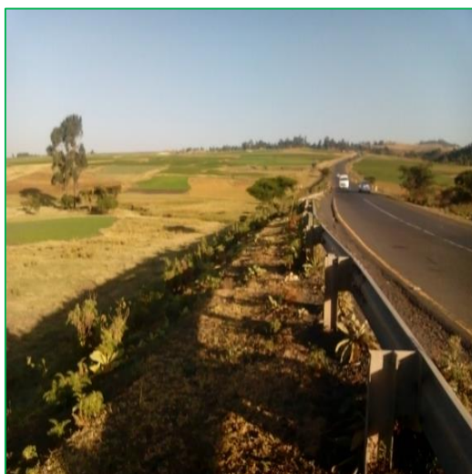
Fig 4.15 Existing road configuration at Wacan Mazoriya
