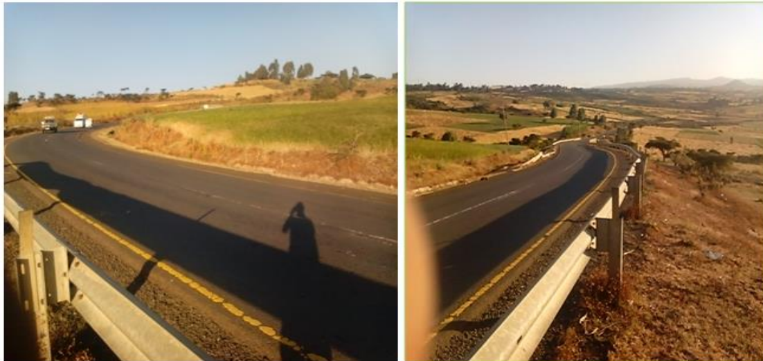
Figure 4.19 Existing Road Configuration at Minini
