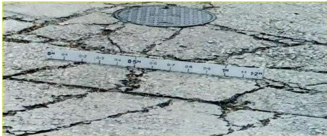
Figure 2.5 Block cracks, [13].
