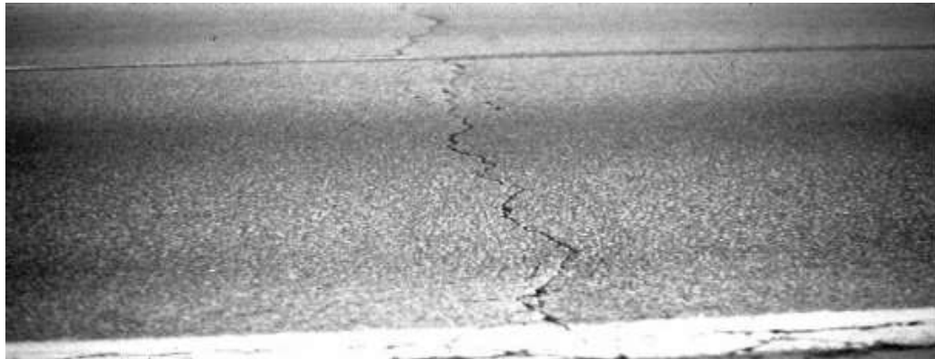
Figure 2.4 Transverse cracks, [17].
