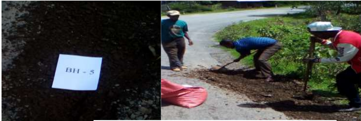
Figure 3.6 Borehole (BH-5) at station 172+300
