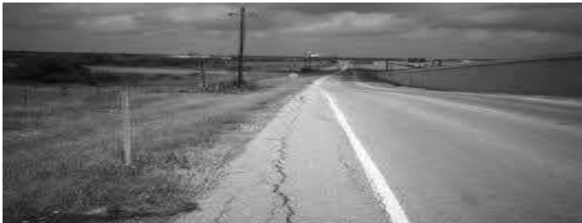
Figure 2.8 Edge cracks, [14].
