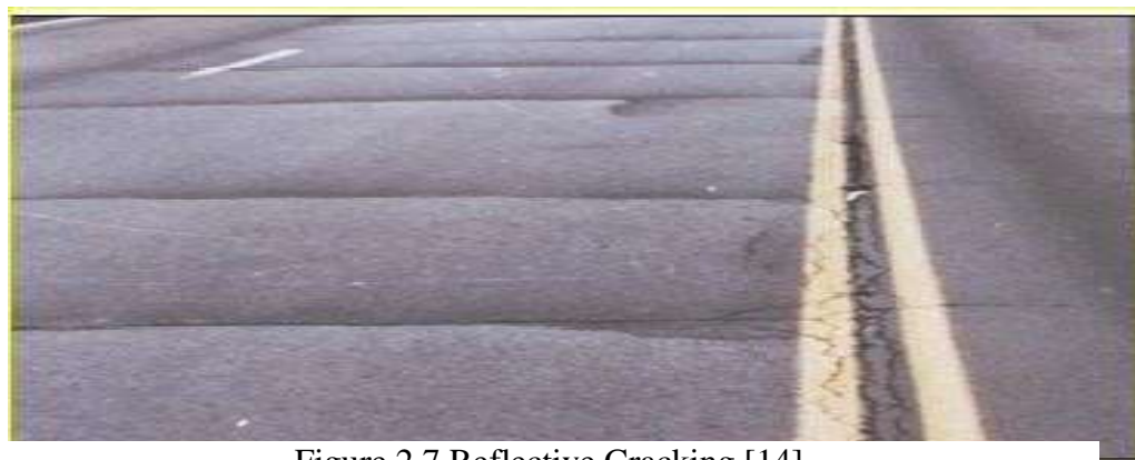
Figure 2.7 Reflective Cracking [14].
