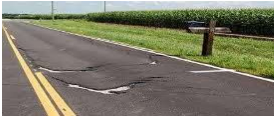
Figure 2.16: Delamination of an overlay, [15].
