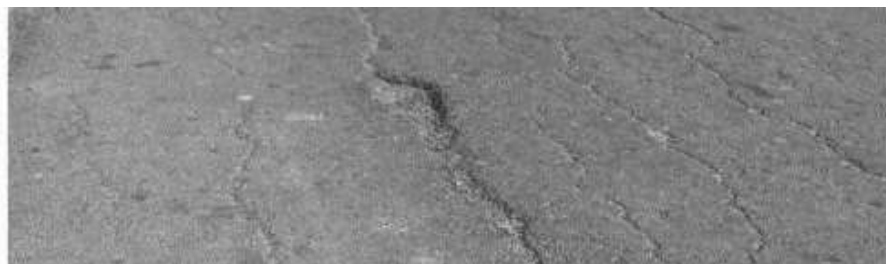
Figure 2.3 Longitudinal cracking, [11].
