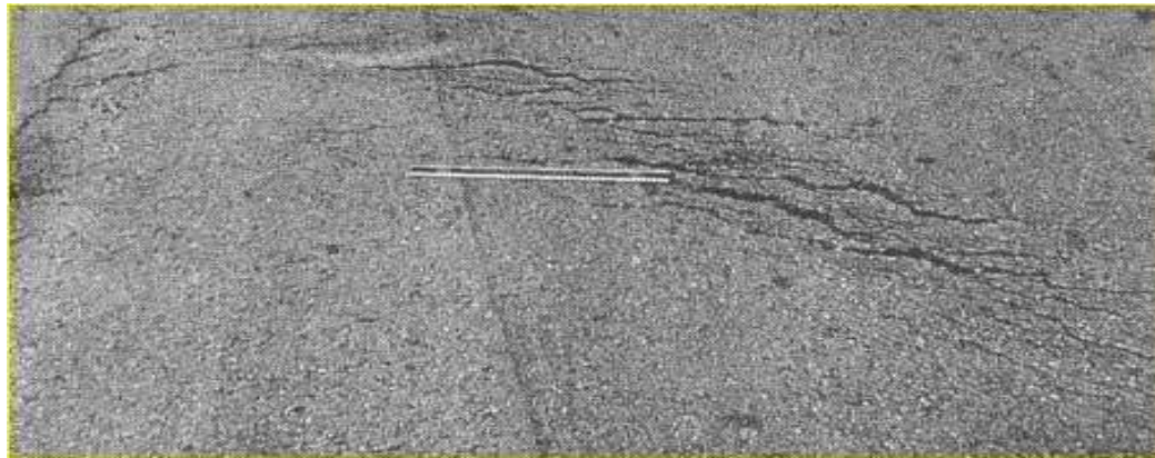
Figure 2.6 Slippage cracks [13].
