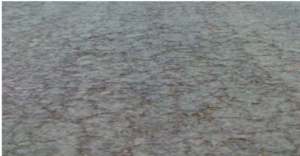
Figure 2.13: Raveling of asphalt surface, [From study road].
