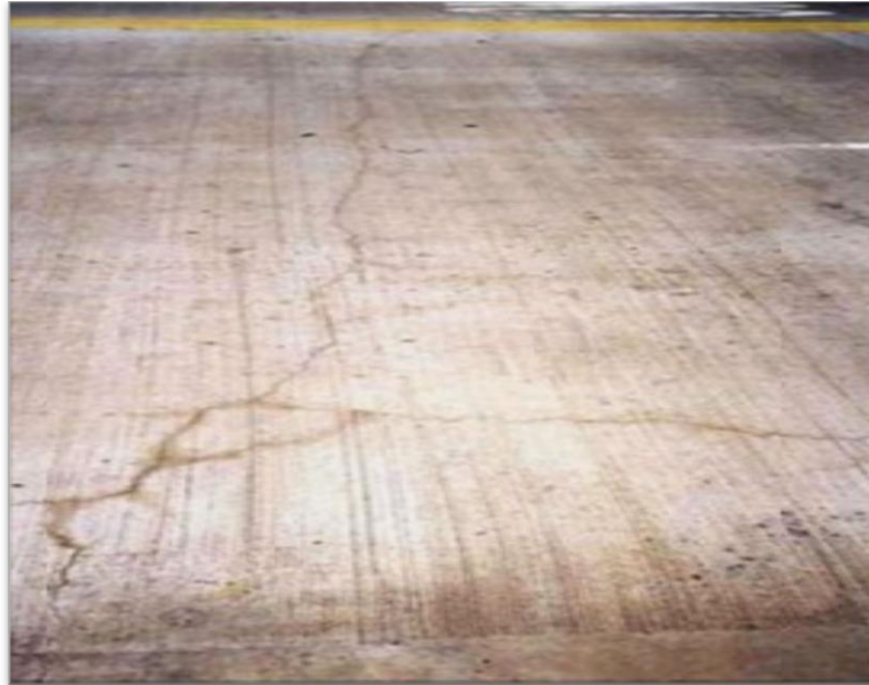
Figure 2.1: Transverse cracking [4]
