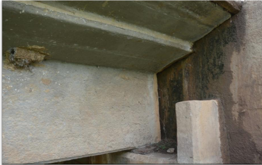
Figure 4.12: Girder end restraint condition
