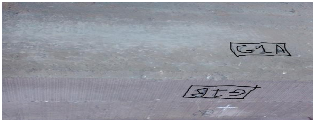
Figure A.1: Surface preparation and coding of exterior girder (G1)
