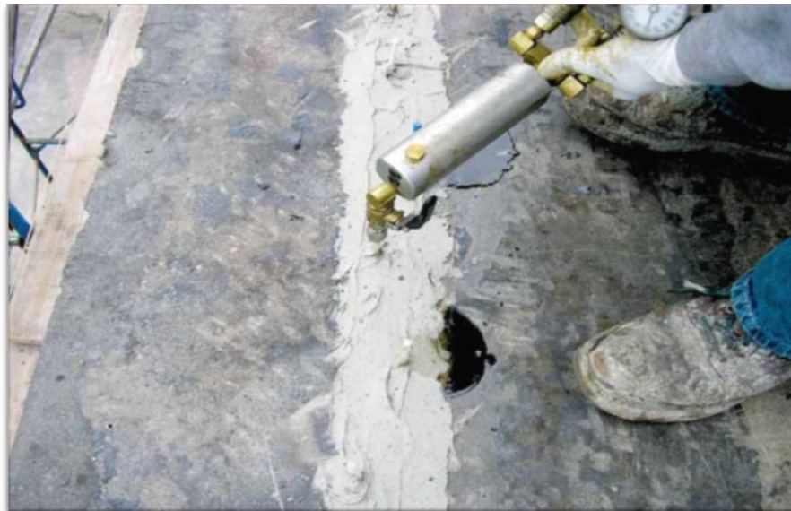
Figure 2.11: Epoxy crack injection [16]
