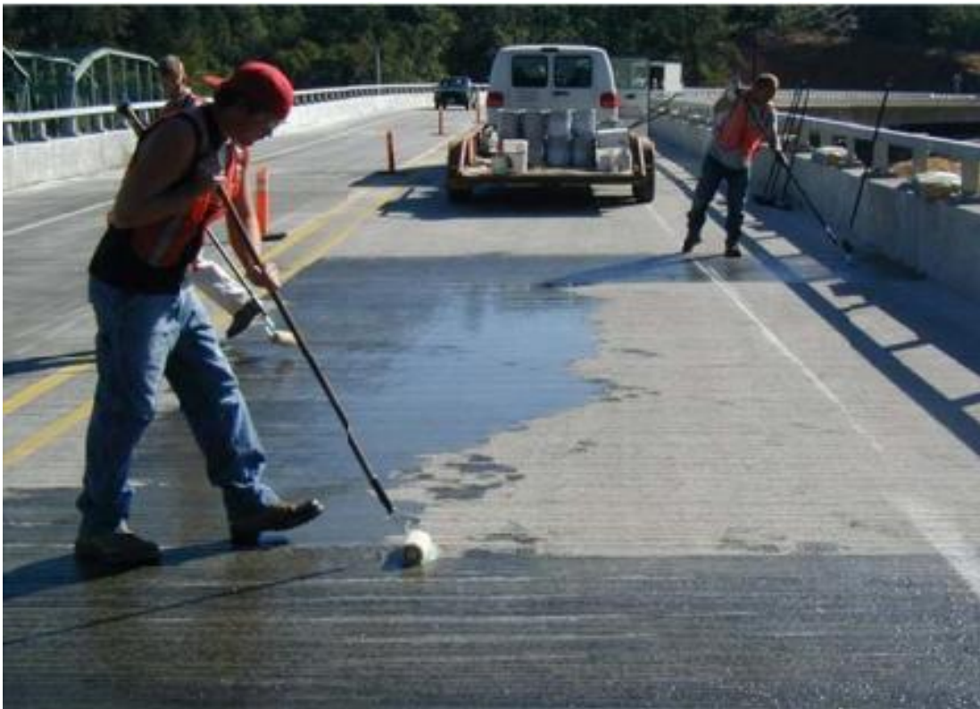
Figure 2.13: Application of a gravity feed repair method [4]
