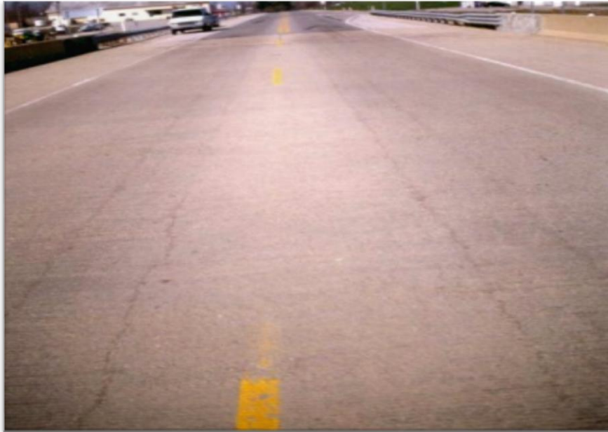
Figure 2.2: Longitudinal cracking [5].
