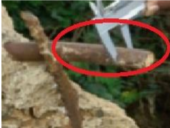
Figure 4.11: Undeformed bare rebar
