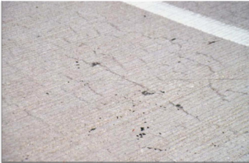
Figure 2.4: Map/Pattern cracking [5]
