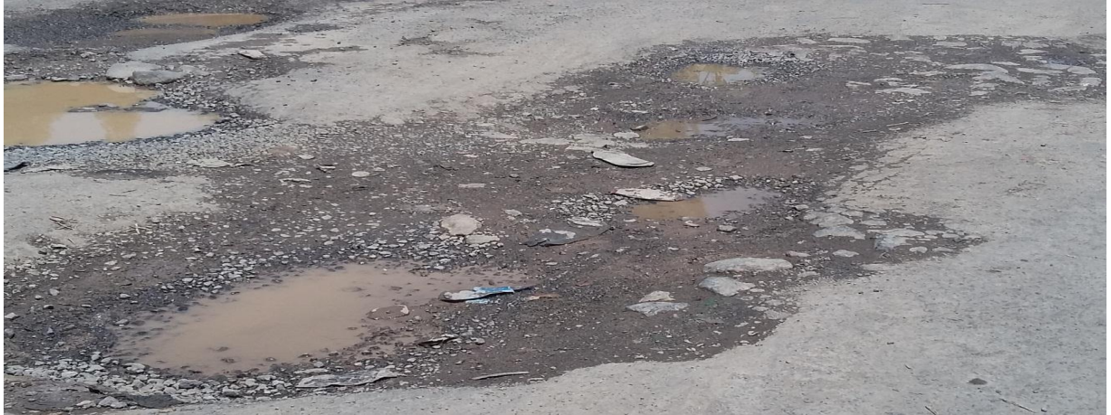
Fig.1.2 Location of the problem of kombolcha-Harbu road
