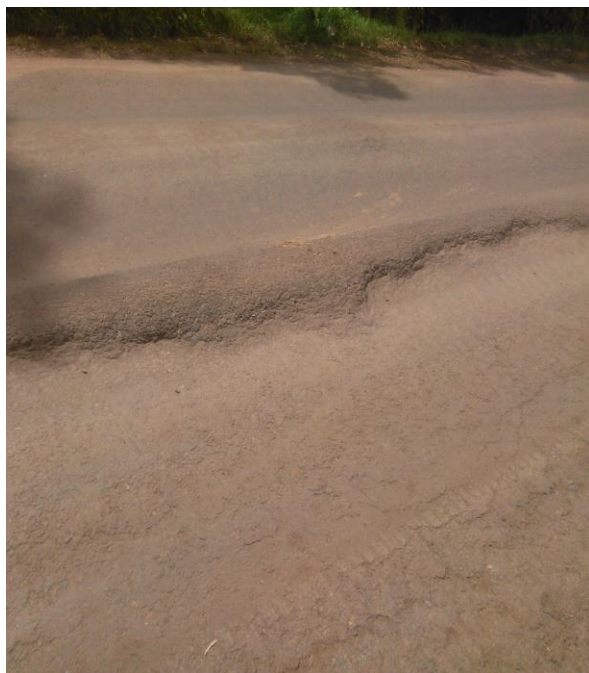
Photo from Bulbulo to Gembe section (39+565)
