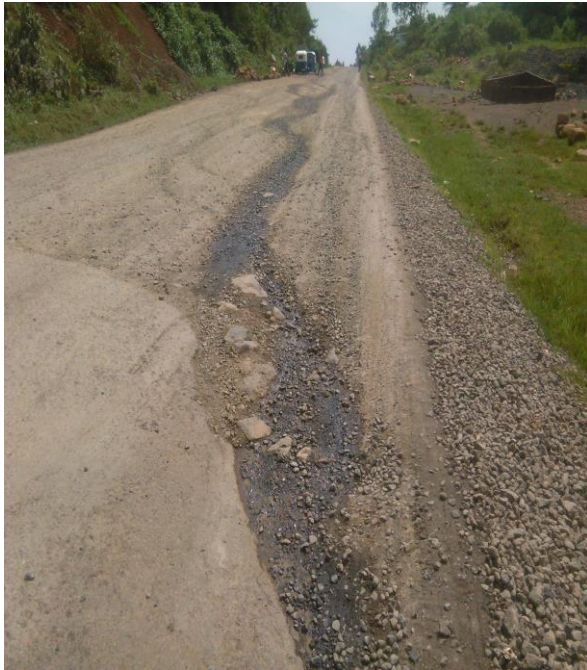
Photo from Bulbulo to Gembe section (38+510)
