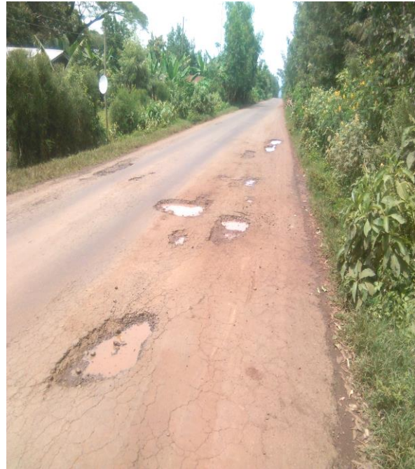
Photo from Bulbulo to Gembe section (39+600)
