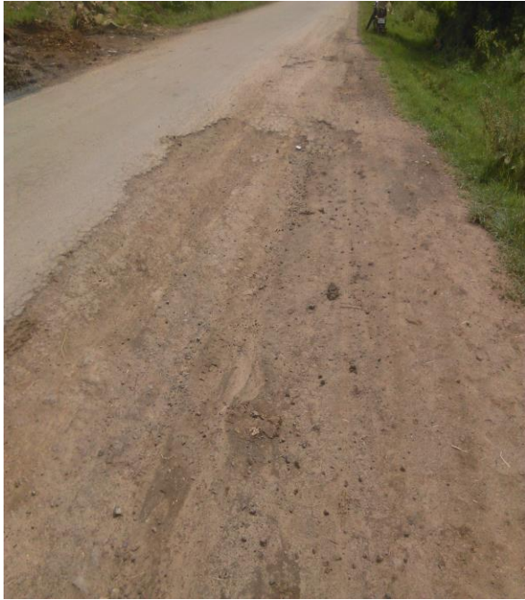
Photo from Dabesa to Yebu section (26+550)
