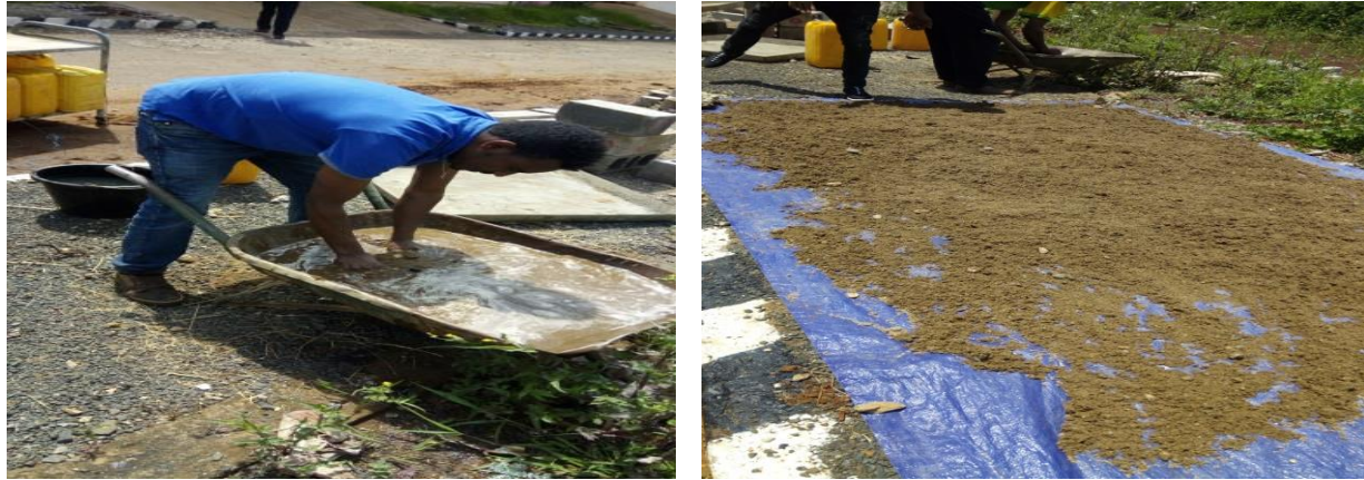
Figure 3. 3 washing of sand to make free of silt and clay.
