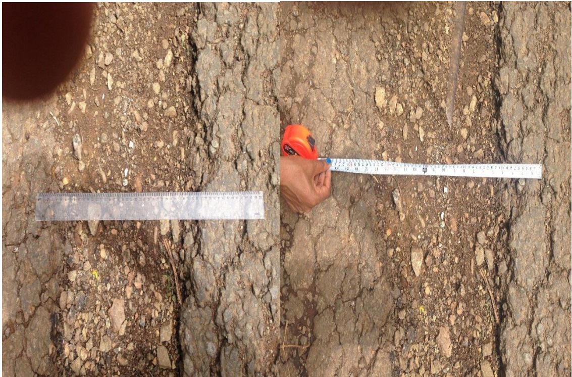
Test pit at station 62+300 before sample collected
