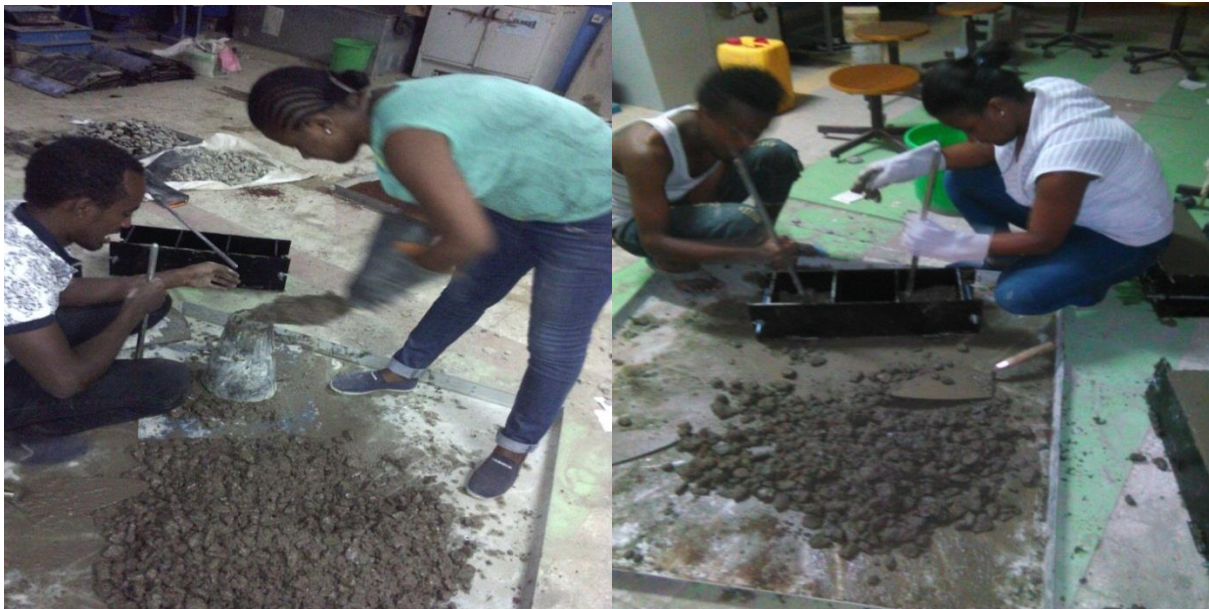
Compaction of concrete by hand for slump test and cube cast
