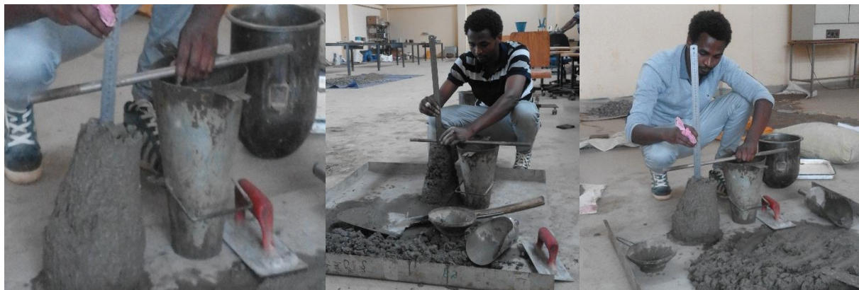
Figure 17: Measuring Slump of Fresh Concrete Mix
