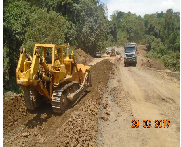
Spreading sub base material using dozer
