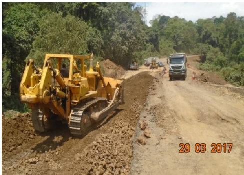
Spreading Sub-base material using dozer
