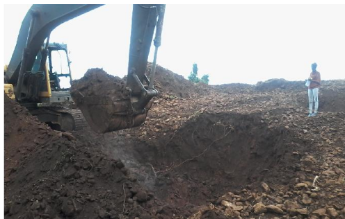
Sub base material production by excavator
