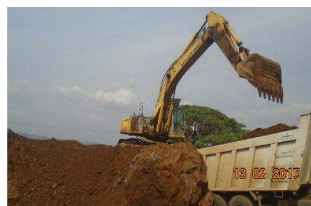
Sub base material production by excavator
