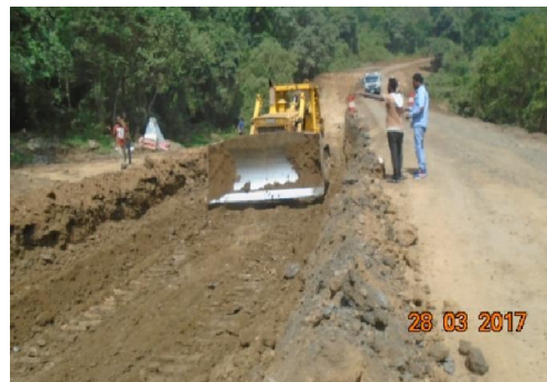
Spreading Sub-base material using dozer
