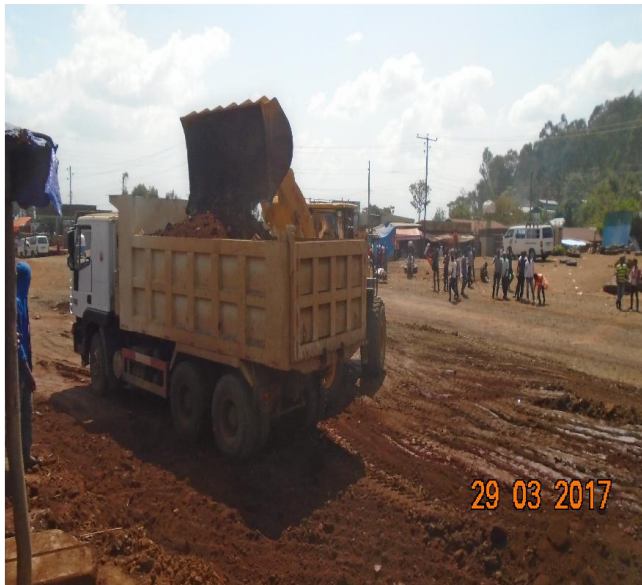
Loading waste material by loader
