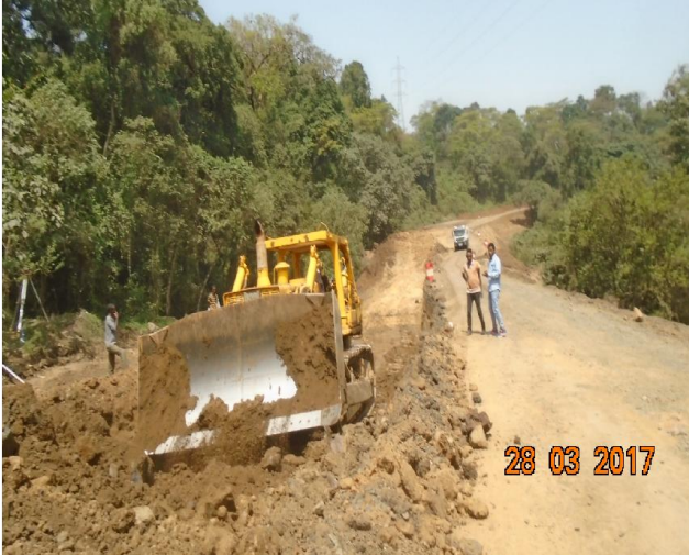
Spreading sub base material using dozer
