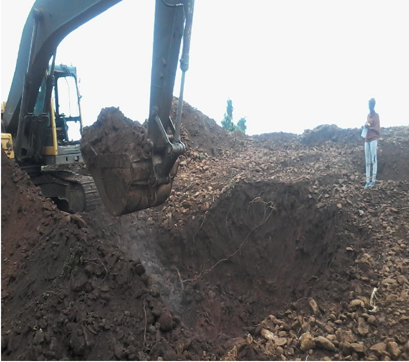
Sub base material production by excavator
