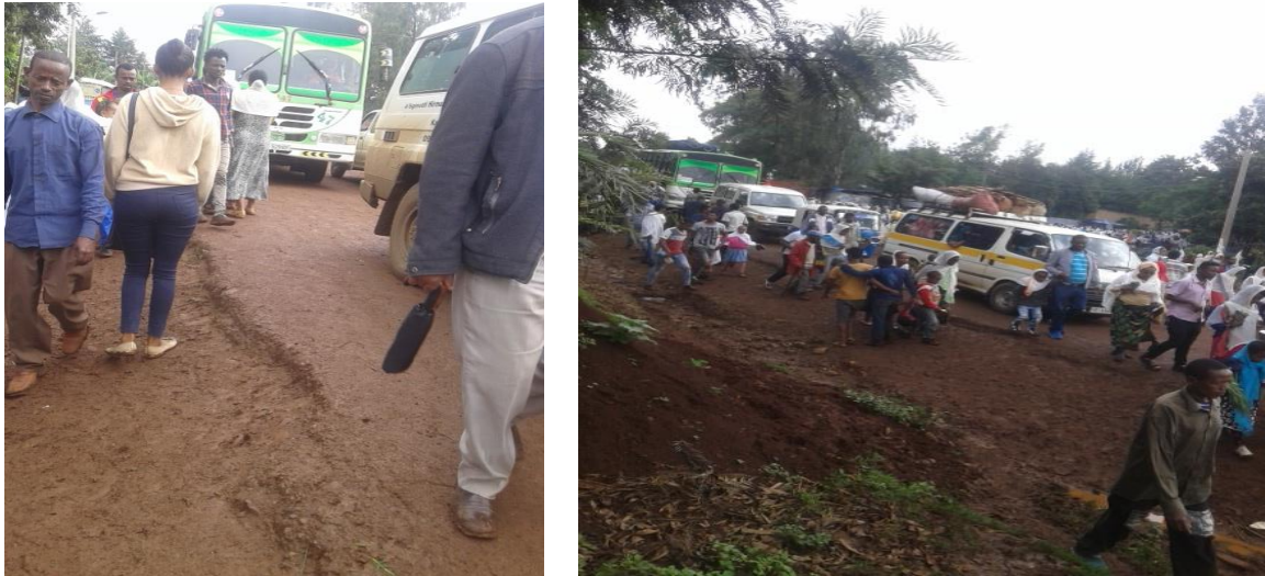
Figure 3. 9 : Field photo with congestion , missing of pedestrian walk way & shoulder at stretch 2
