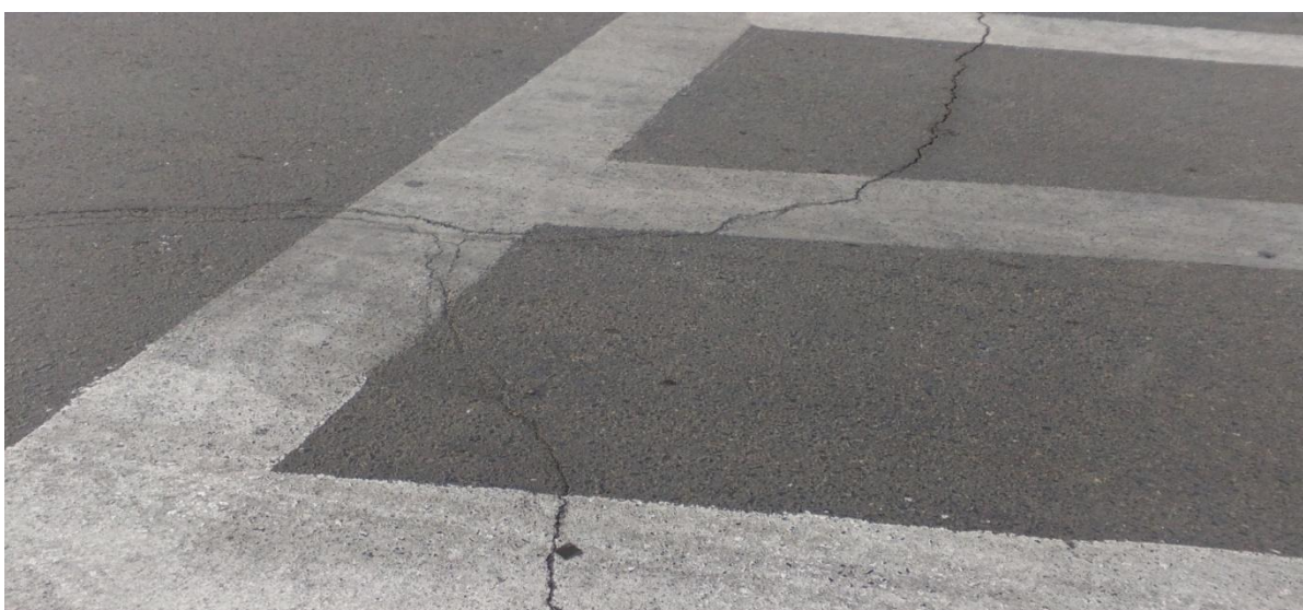
Fig.4.5: Photo: National Theatre 2 site: after 8 months of geogrid reinforcement.
