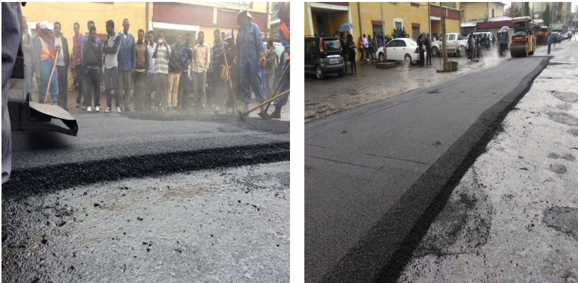
Fig 3.12 Photo: Placement of 40mm overlay at the Gandhi Hospital Site
