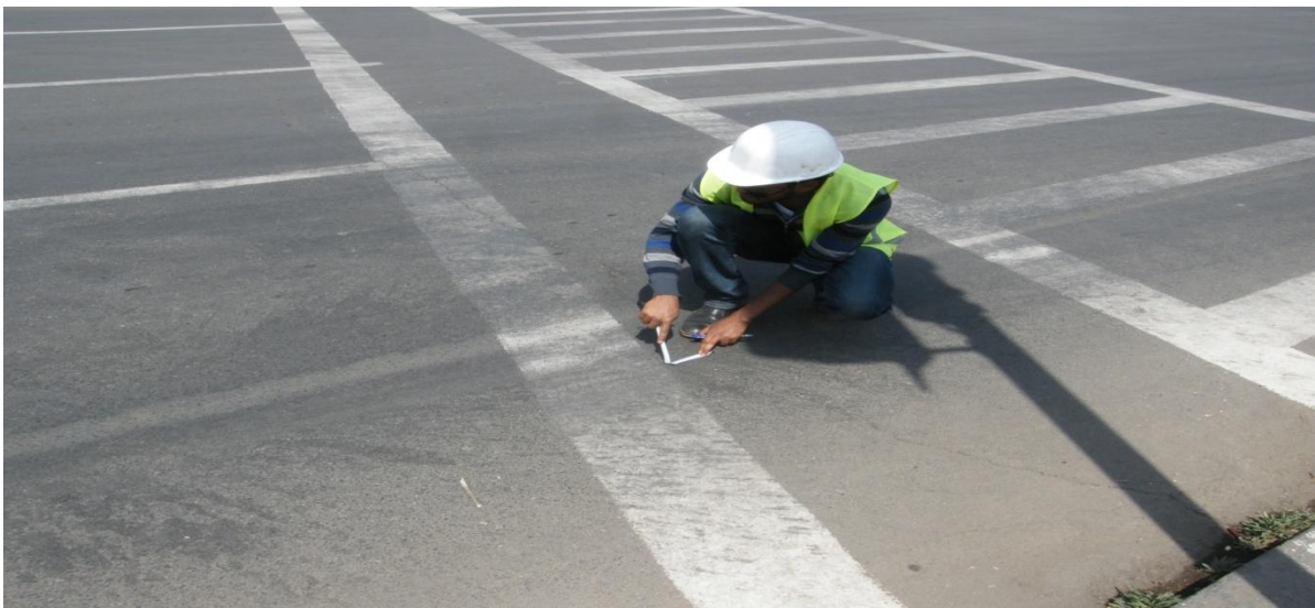
Fig.3.7: Photo: Taking of measurements at the National Theatre site
