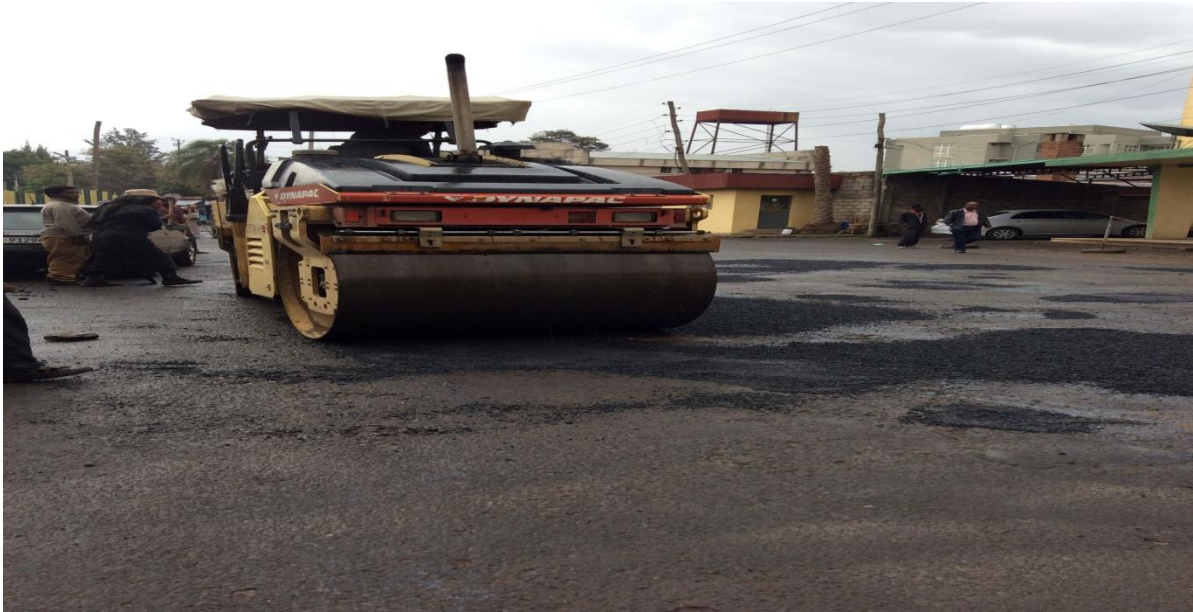
Fig.3.5: Photo: Leveling and compacting of treated areas using a roller compacter
