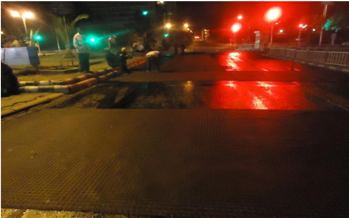
Fig. 3.11, Photo: Transverse direction of Geogrid installation at National Theatre 2 site
