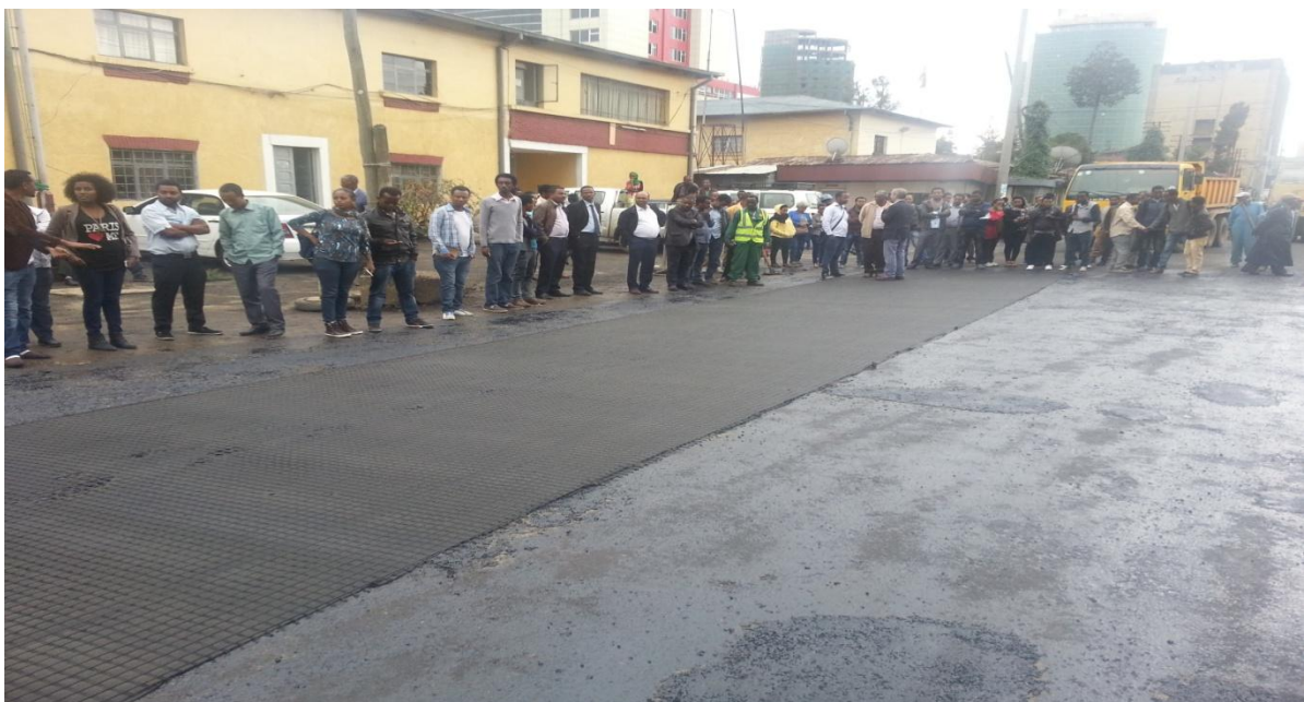
Fig. 3.10, Photo: Longitudinal laying of Geogrid at the Gandhi Hospital site
