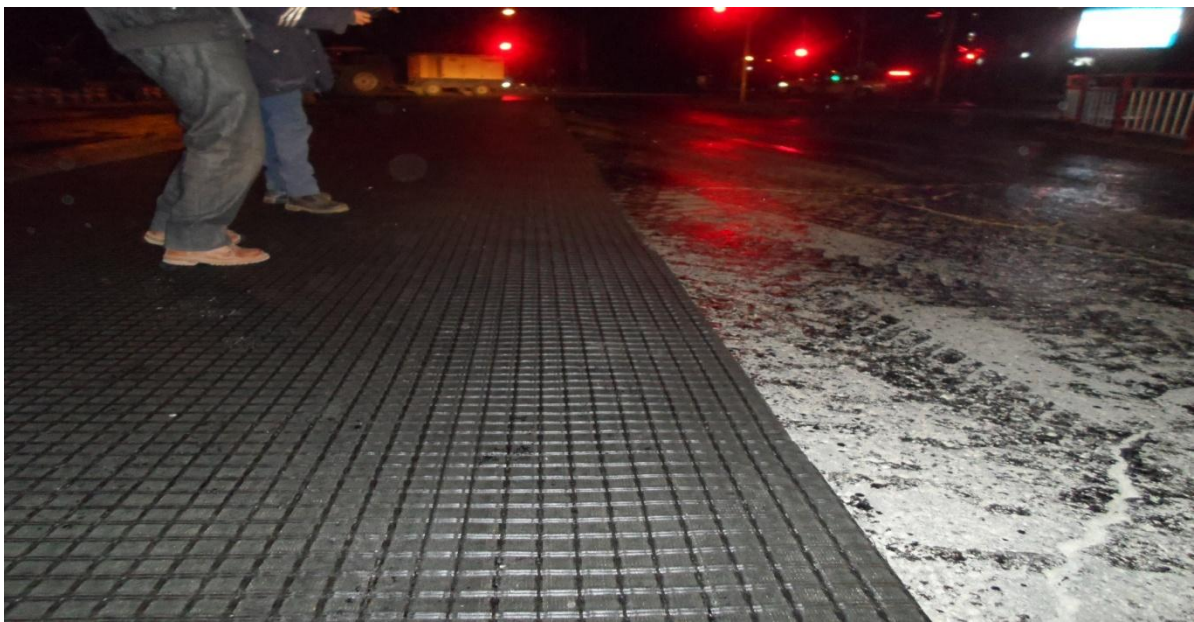
Fig: 3.9 Photo: Longitudinal laying of Geogrid at National Theatre 1 site:
