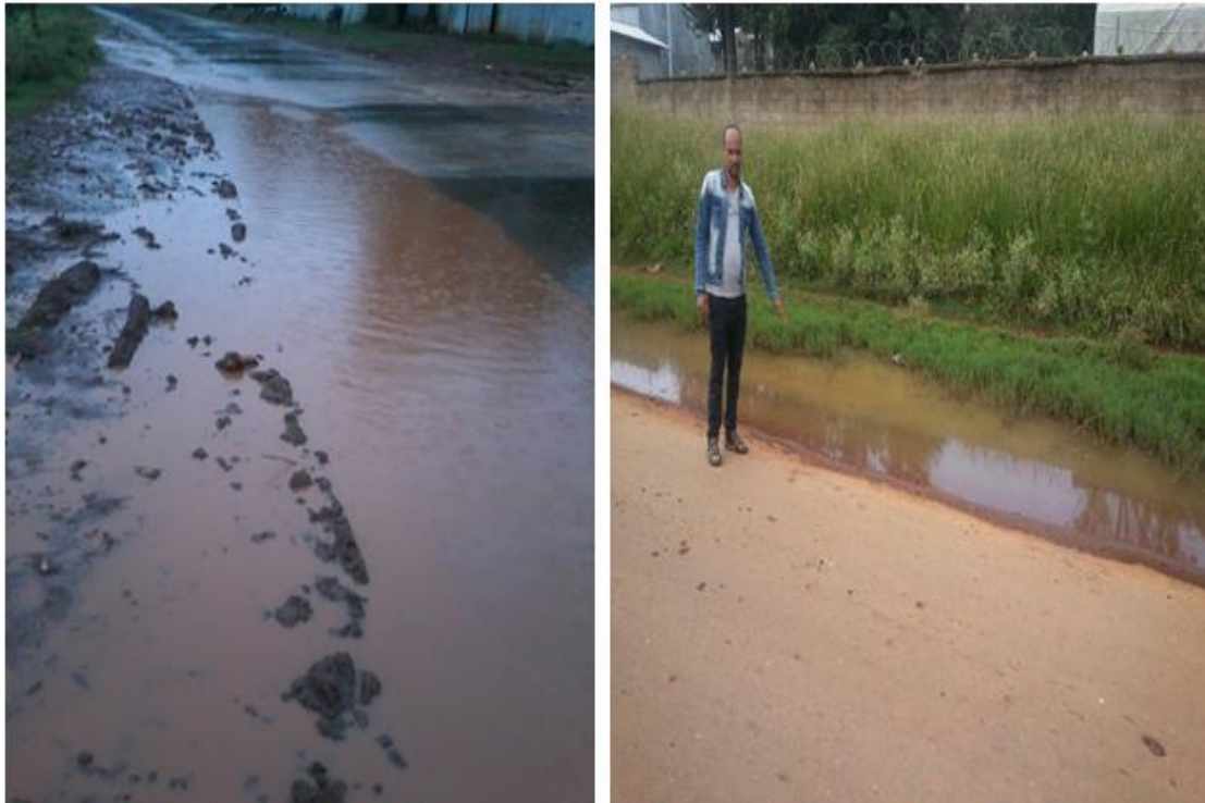
Figure 4.16: Taken June 12/2016 Water ponded along the study area road at a Jimma town near the back of Agricultural and veterinary medicine college fence.
