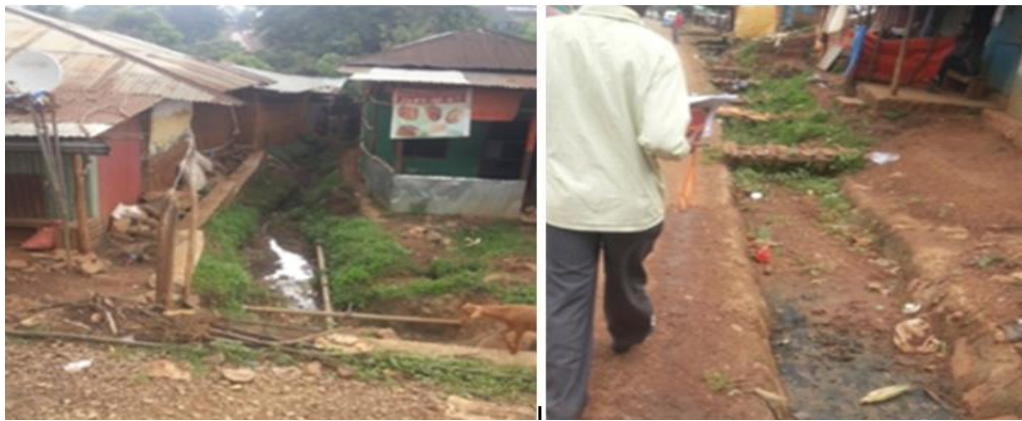
Figure 4.19 Taken June 12/2016, Blockage by silt soil, garbage and upland houses in yebu town along the study area
