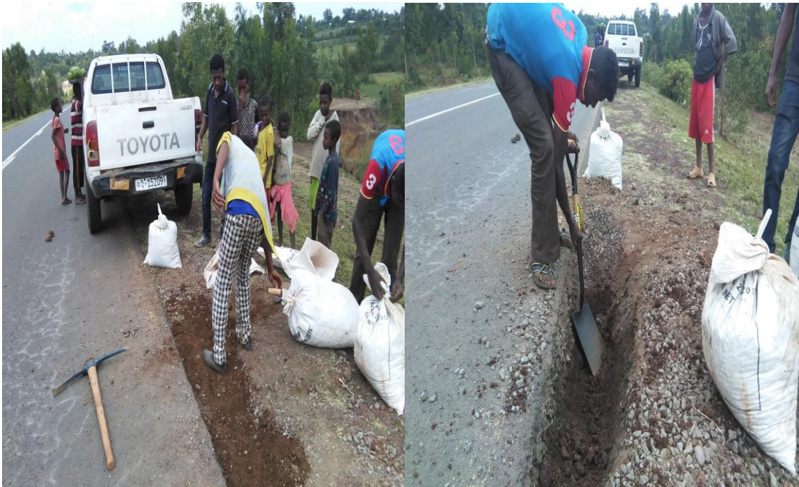
Figure 3-11: Repairing and replacing for excavated pavement layers at section Alaba-Mazoria
