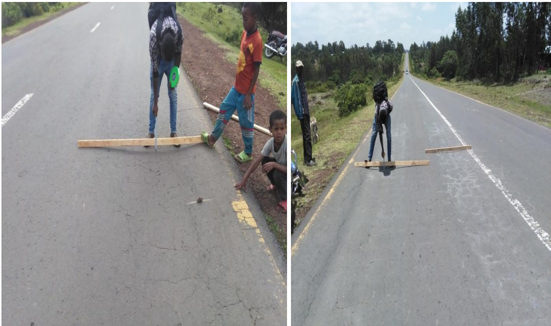
Figure 3-4: Shows the pavement condition surveys on sub section road Buge to Boditi.
