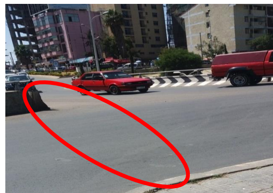
(b) Inadequate Entry Lane
