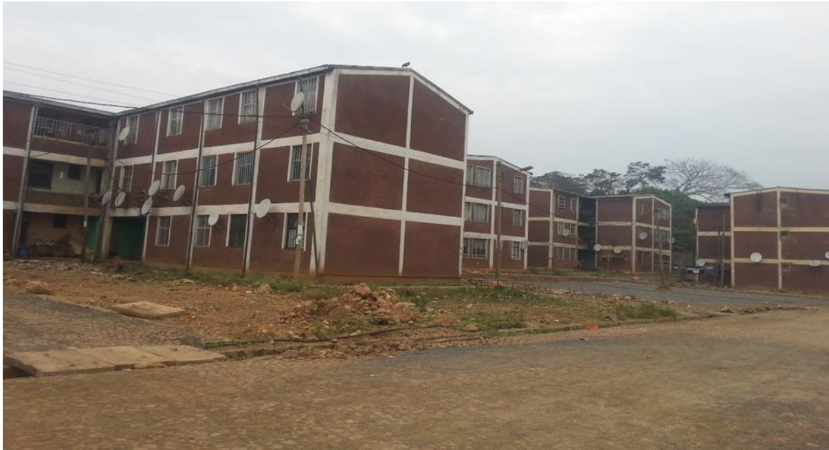
Figure 1. A Picture from Kella condominium Site in Jimma town, Ethiopia
