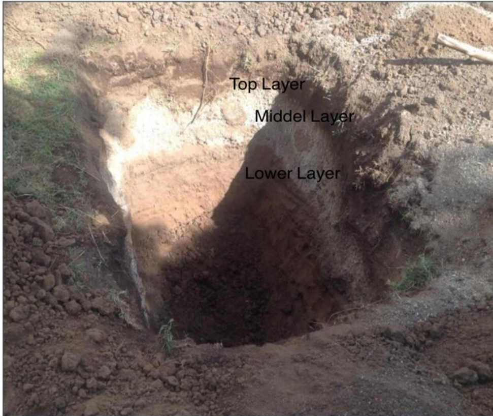
Figure3.1:- photo of general soil layer of excavated test pit
