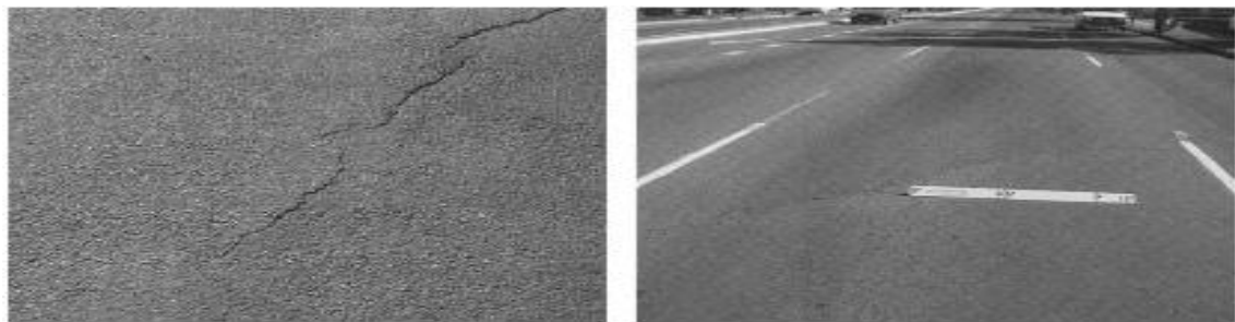
Figure2.9: Diagonal Cracks in flexible pavements (Source: Zahidul, 2006).
