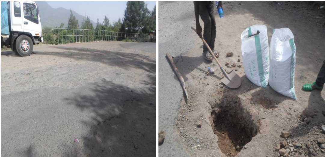
Figure 3.3 Representative Raveling Damage and their sample (20/09/2008)
