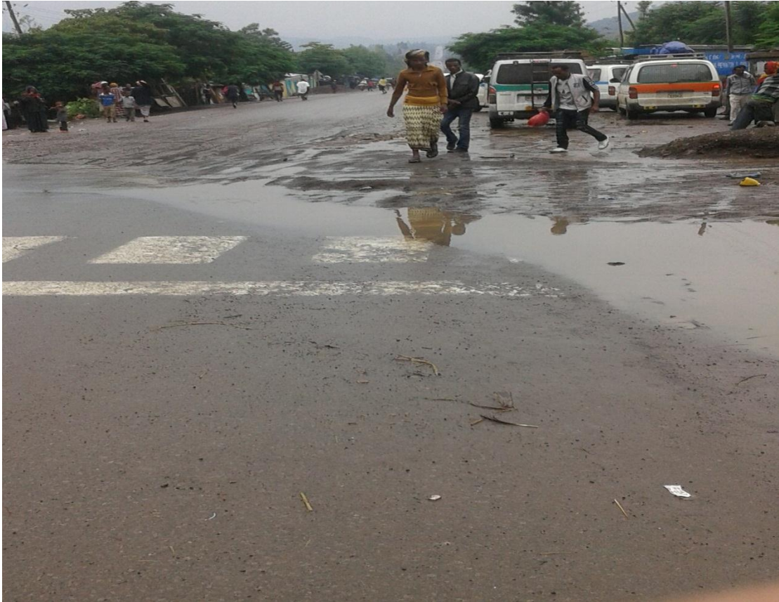
Figure4.16: Drainage problem in Harbu town
