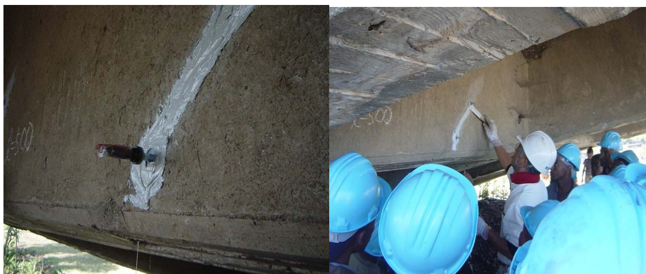
Figure 6: Injection with flexible filler
