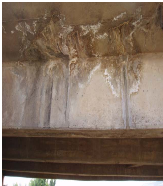
Figure 8: Water leakage and deteriorations
