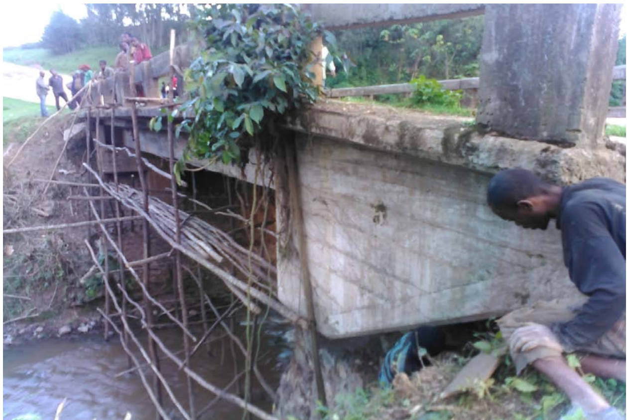
Figure 9: Scaffolding during measuring and quantifying of defects
