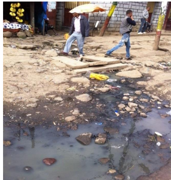
Fig 3.6 d) Inlet operate with problem
