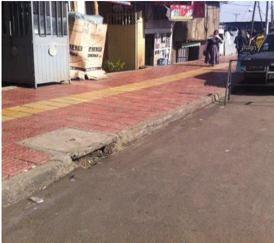
Fig 3.5 a) Inlets in good condition
