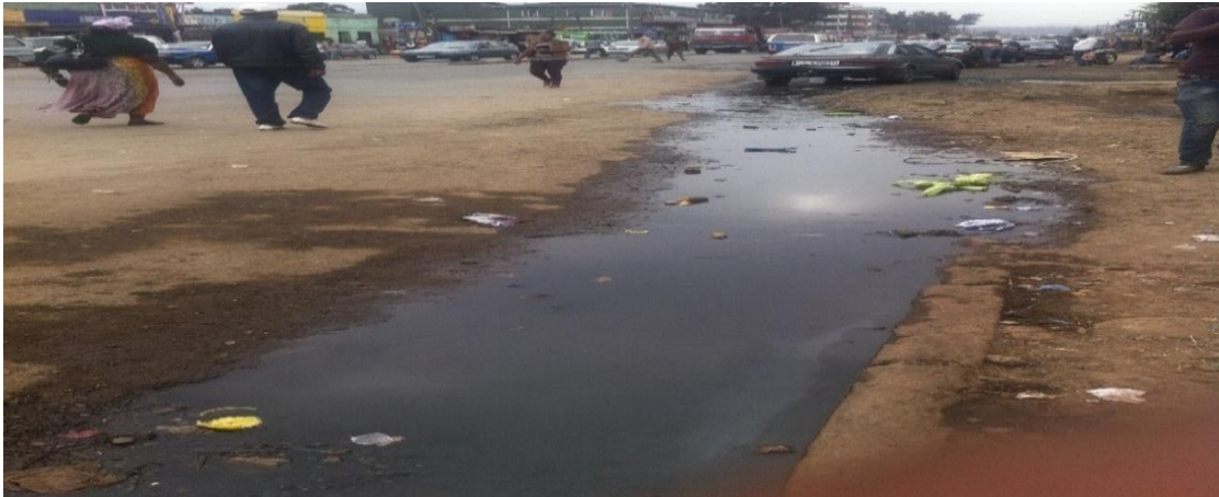
Figure 2.1 side drain (January 2017)
