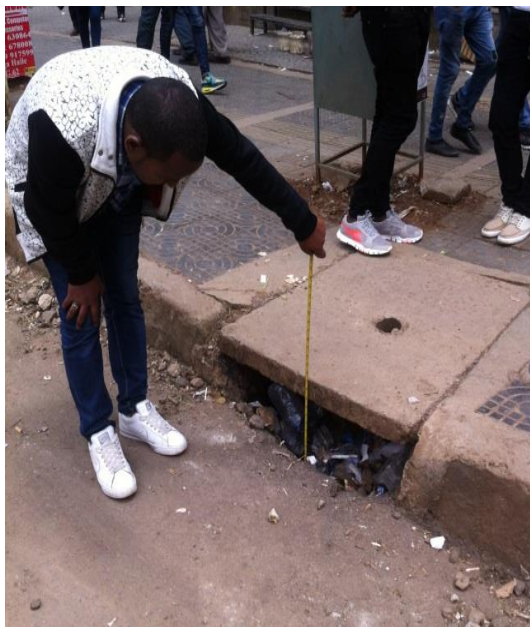
Fig 3.6 a) Inlets in good condition
