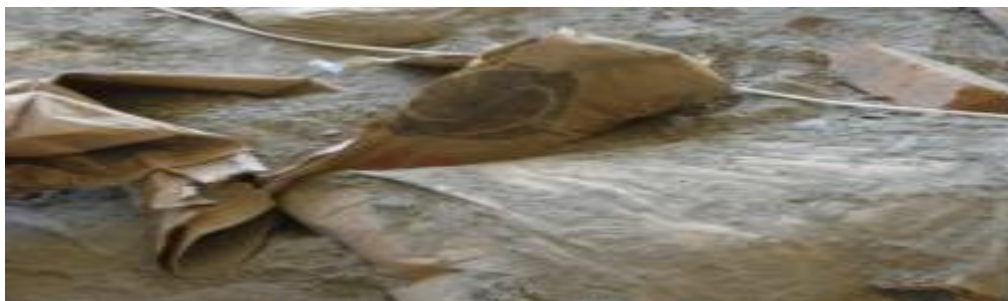
Figure 4-14: Unsuitable stock location of cement
