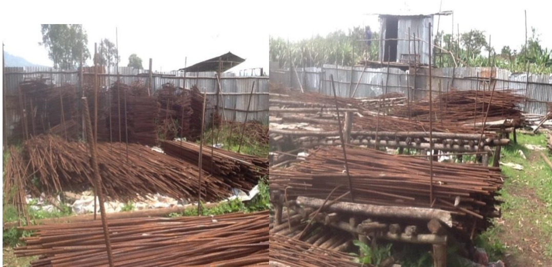
Figure 4-16: Good Storage and handling of Steel Reinforcement on construction sites
