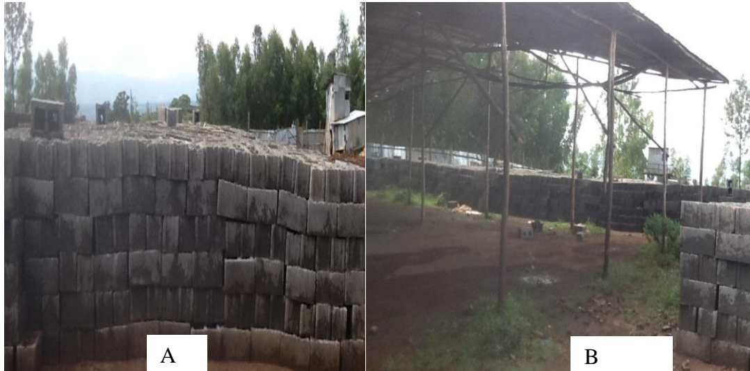
Figure 4-9: Good handling of HCB during storage at VARNERO on site
