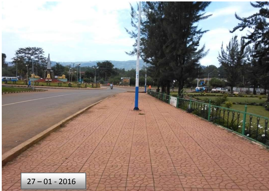
Figure 4.10 walkway with good continuity (Around Farmid )
