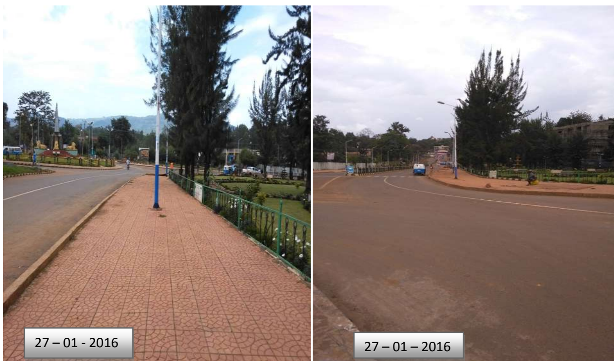
Figure 4.13 Walkway with good visibility ( Around Hermata)
