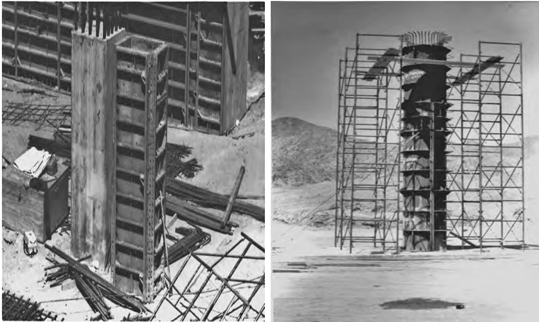
Figure 2.8: Modular steel form for rectangular columns and round-column forms with access scaffolding in preparation (David, 2007).
