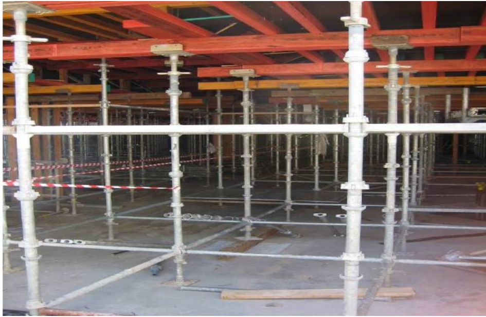
Figure 2.14: Typical support scaffold (Tayakorn and Rasmussen, 2009).
