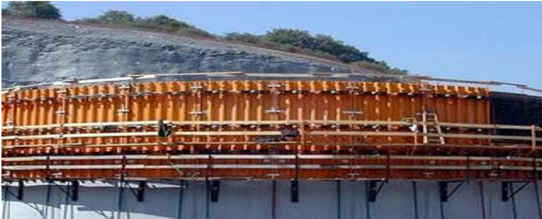
Figure 2.2: Steel Formwork (Chirag, 2011).
