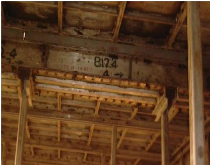
Figure 2.3:Mivan Formwork (Kumathekar and Swapnali, 2007).
