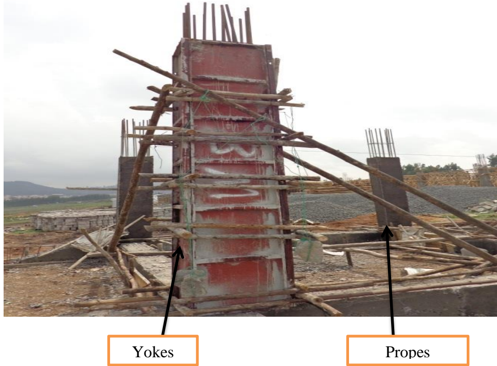
Figure 4.5: Column formwork construction systems using steel at legetafo site
