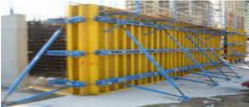
Figure 2.7: Vertical forming system (David, 2007).
