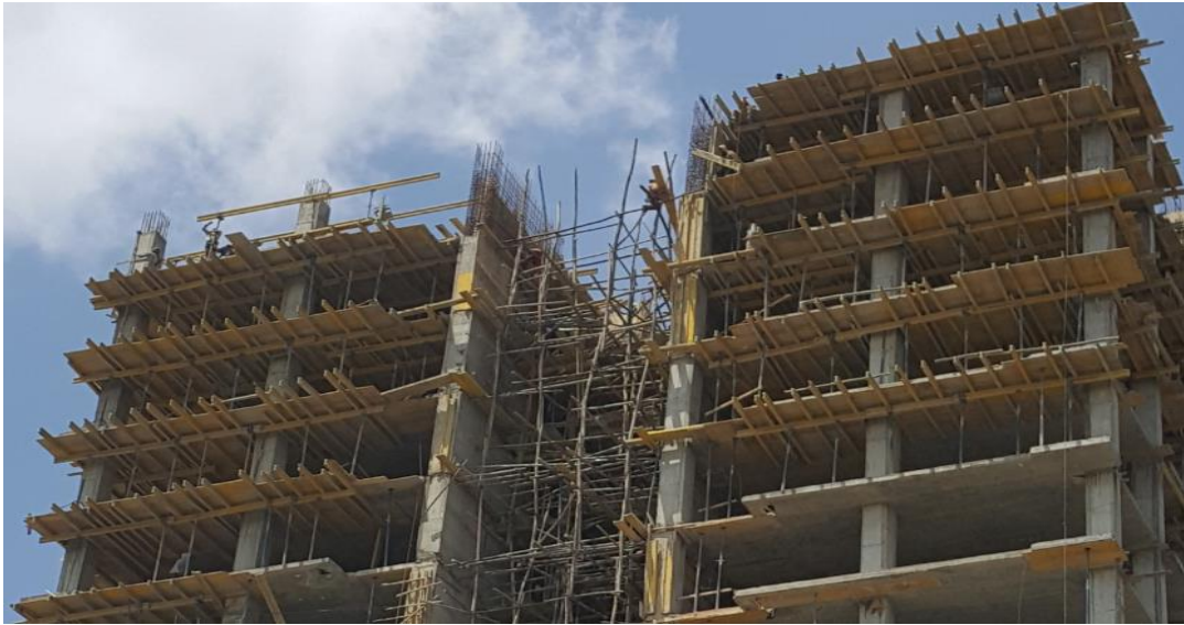
Figure 4.2: Yellow timber formwork at megenagna site
