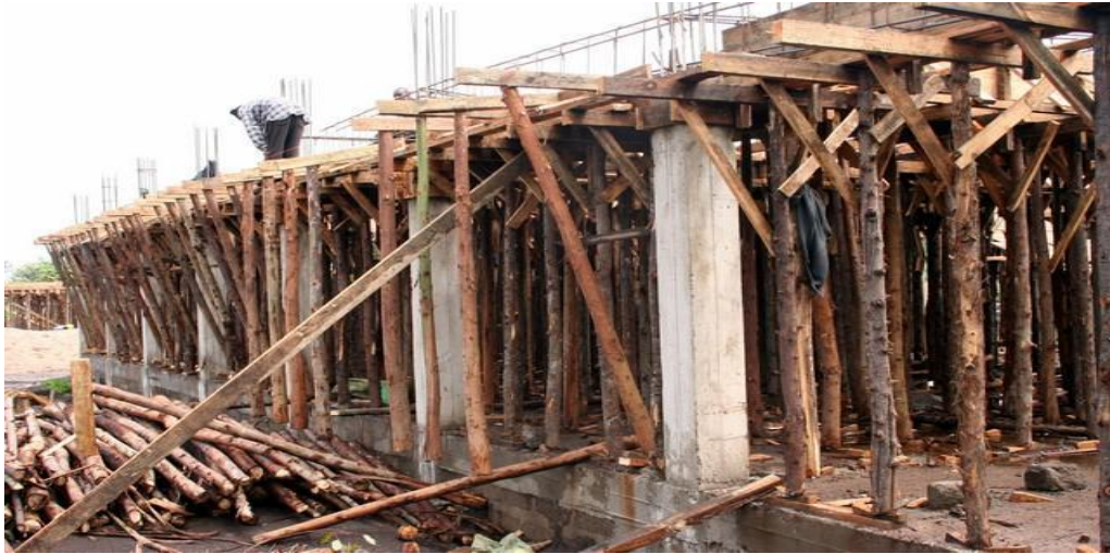
Figure 2.9: Slab formwork (UNITEC, 2009).
