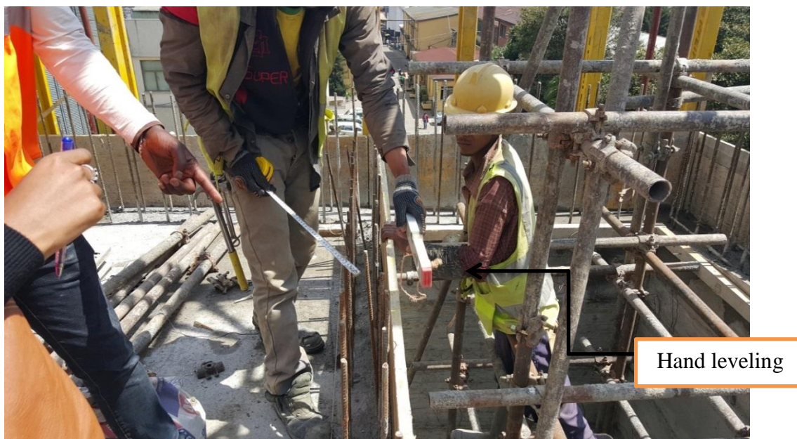
Figure 4.8: Horizontal alignments checking at Mexico site
