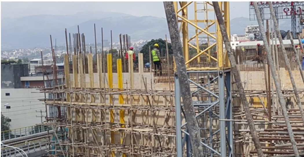
Figure 4.16: Steel scaffolding at Mexico site
