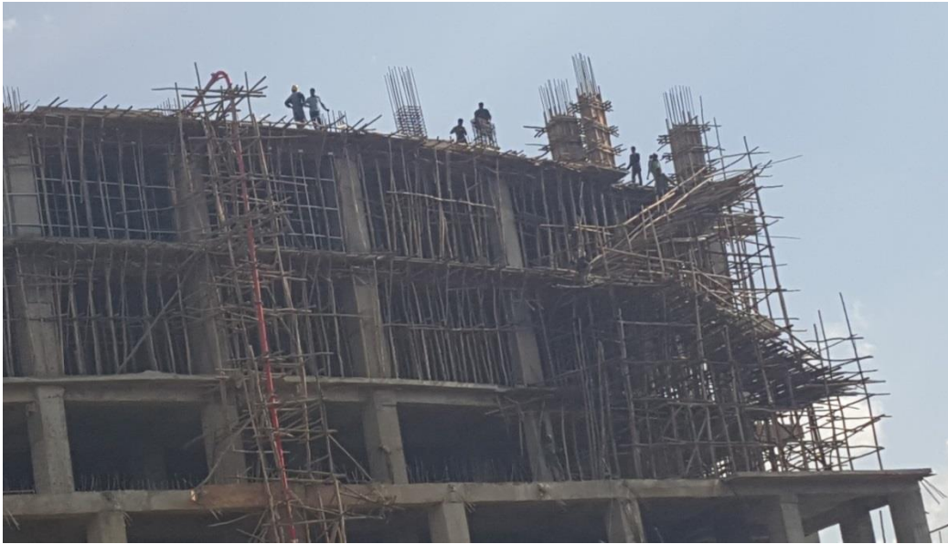
Figure 4.15: Timber scaffolding at legetafo site.
