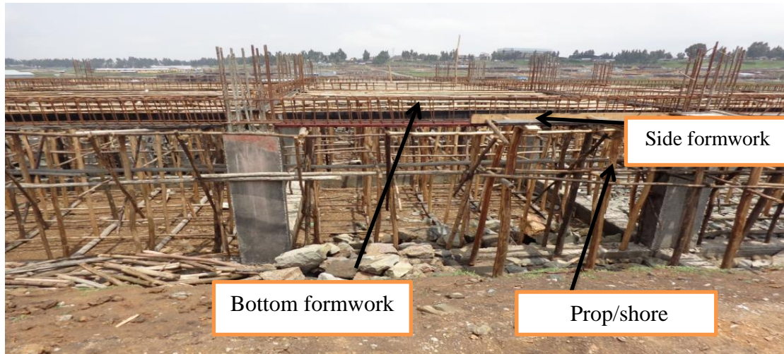
Figure 4.7: Slab and beam formwork at legetafo site.
