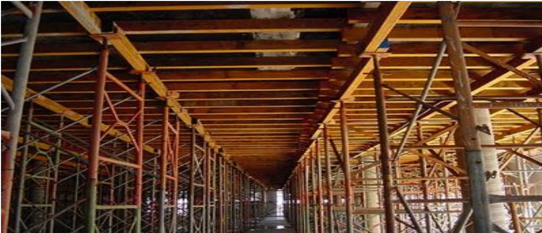
Figure 2.1: Wooden formwork (Chirag, 2011).
