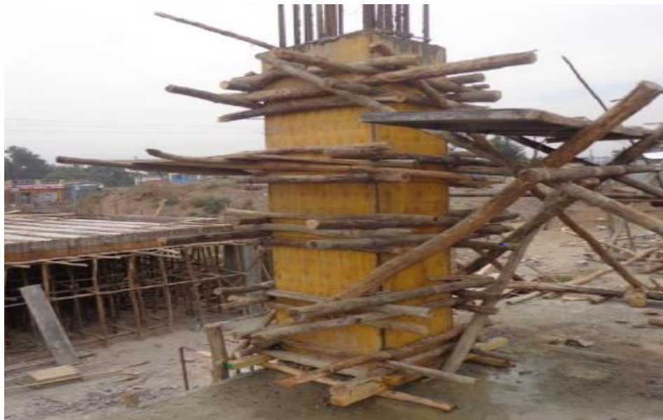
Figure 4.6 : Column formwork construction systems using timber at Paulos site
