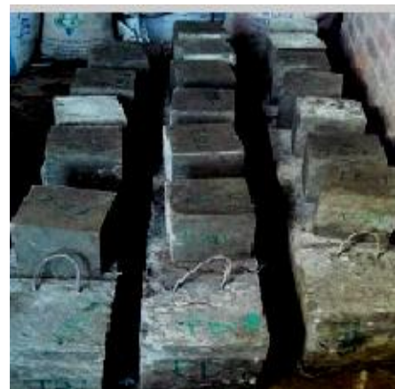
d) removal of formwork
