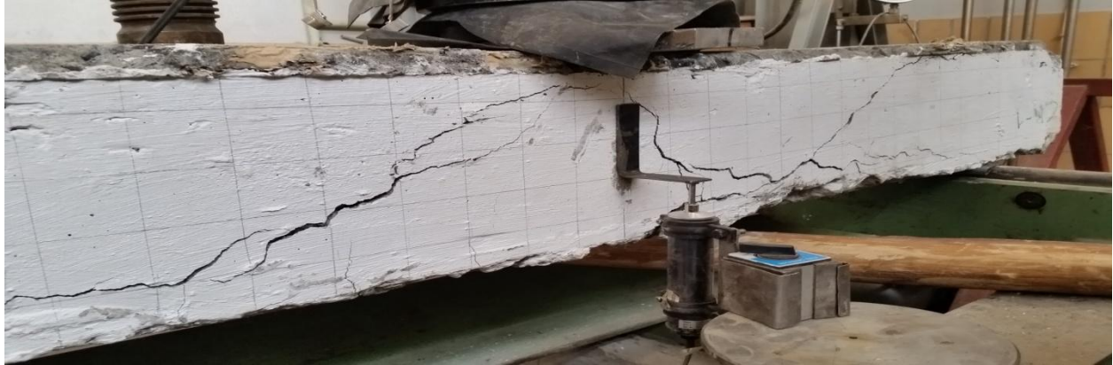
Final failure mode
