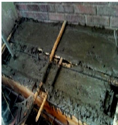
c) Casting and compaction of concrete
