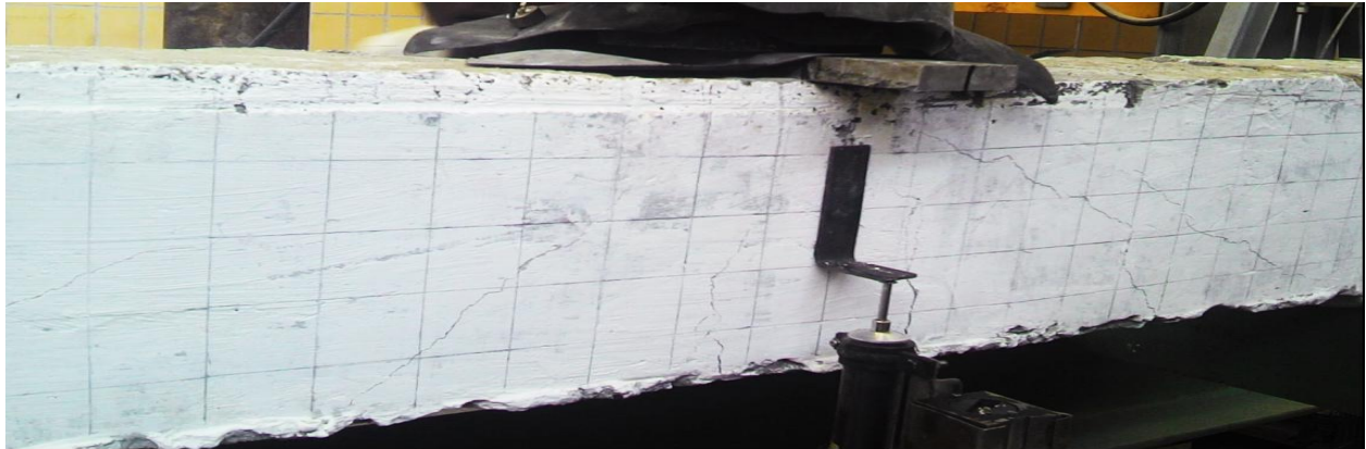
Figure4. 7 Cracks propagation for TB-1
