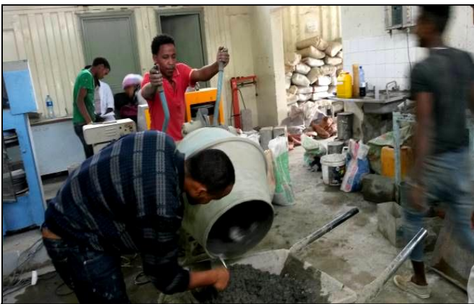
Figure 3.6: Preparation of Concrete Mix
