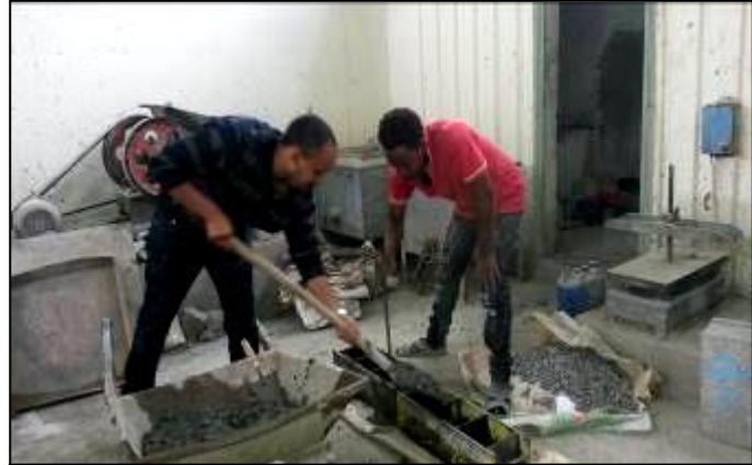
Figure C.1.14: Concrete Casting and Compacting
