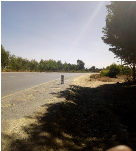
Figure 4.11 Inadequate shoulder width
