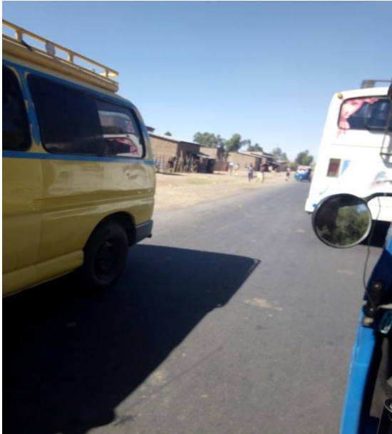
Figure 4.22 No center line between the two directions
