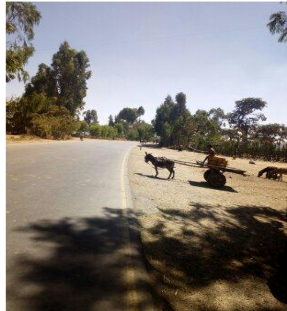
Figure 4.23 No zebra crossing
