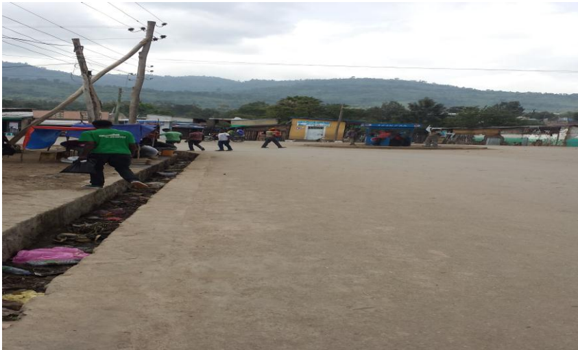
Fig 4.17 No center and edge line and zebra crossing near round about
