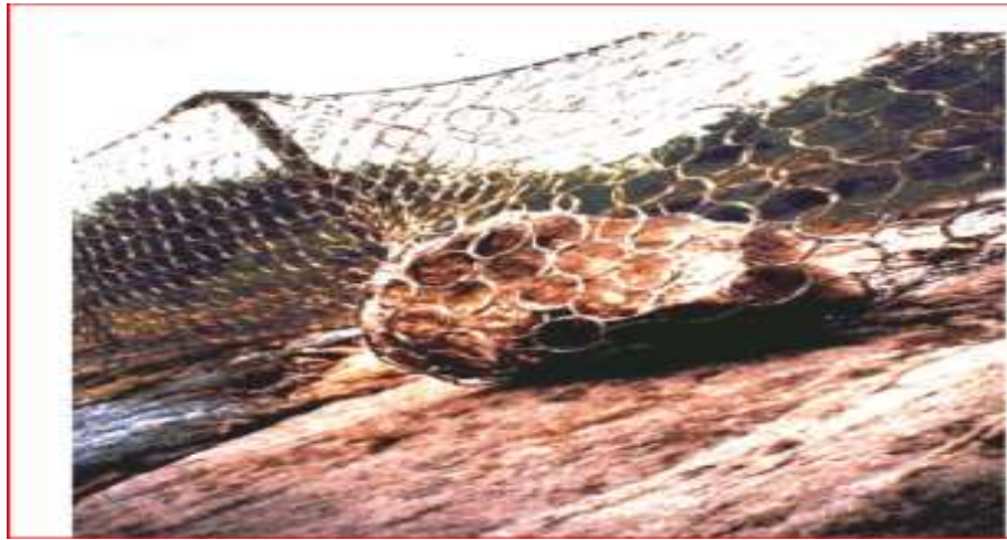
Figure 2.4 Geo-brugg ring net restraining after (Spang, R.M., Soñner, T., 1995)
