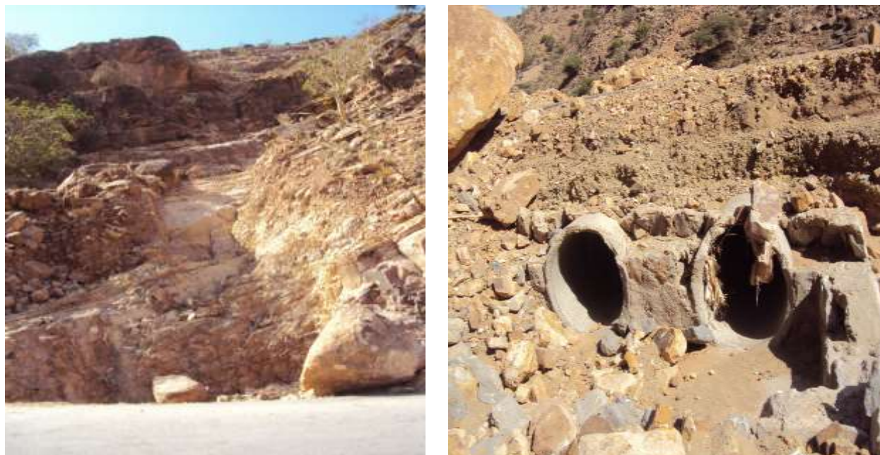
Figure C1.1 Blocked culverts
