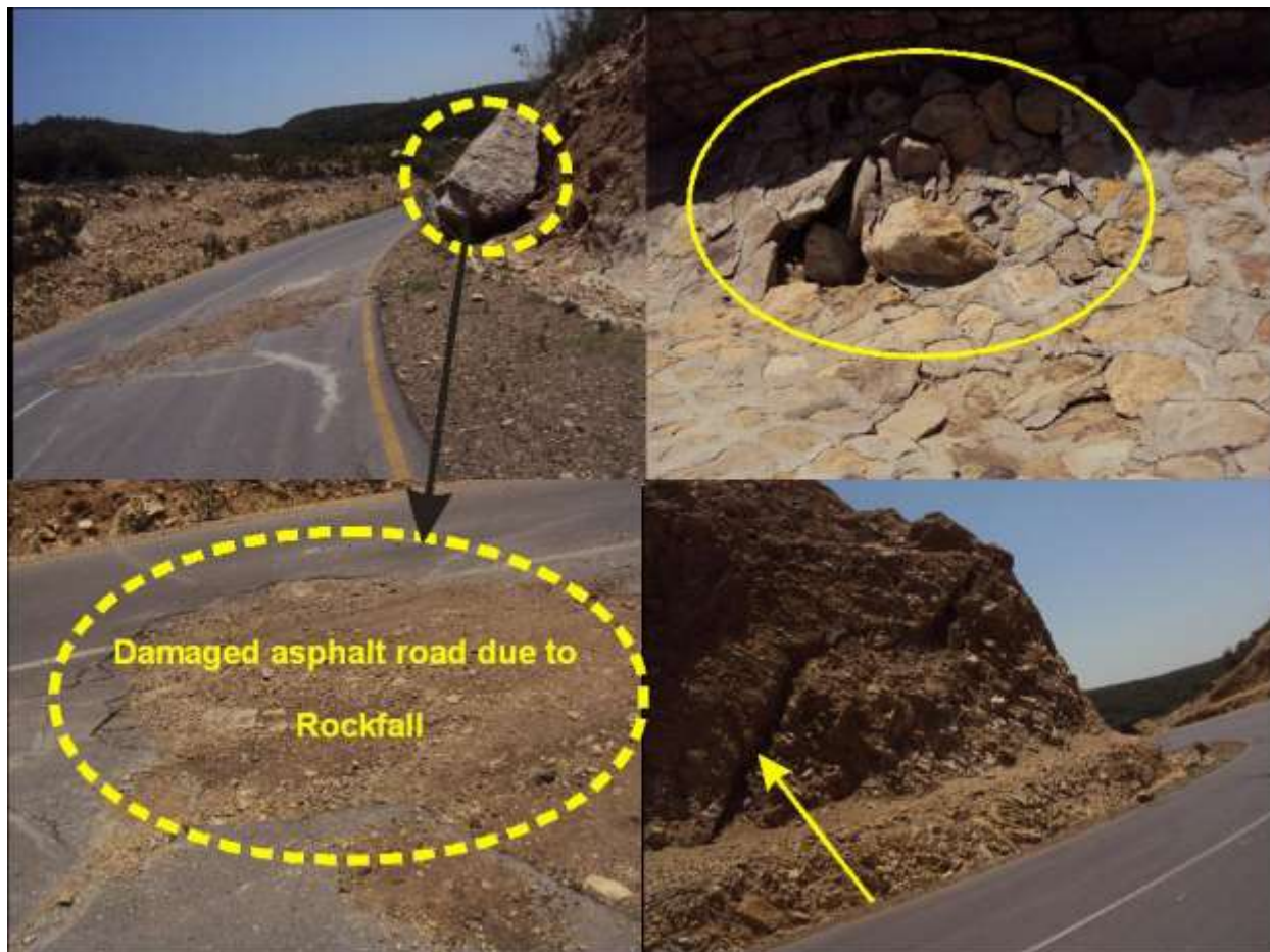
Figure D1.4 Cracked slope
