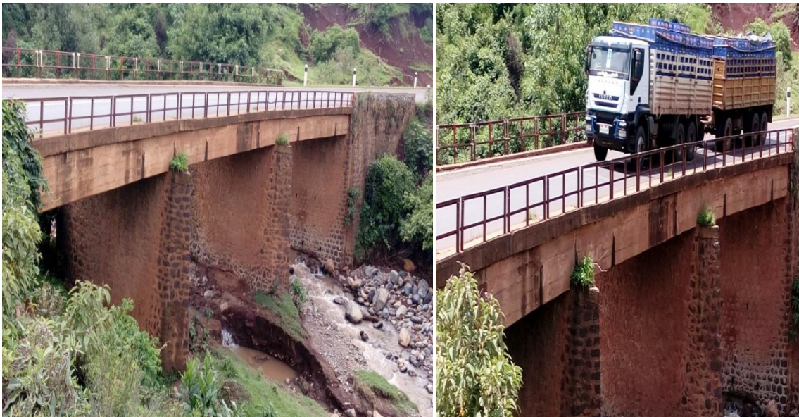
Figure 3.1 Side View of Oda Bridge
