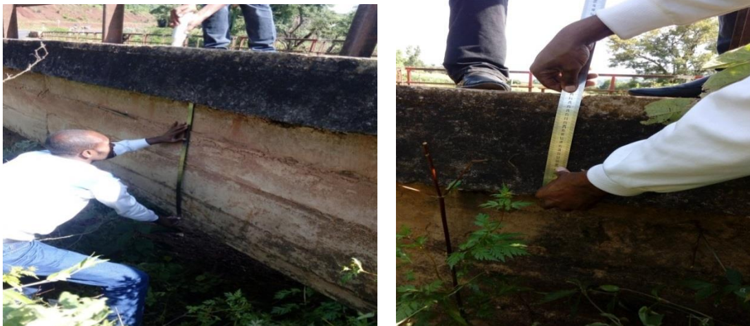
Figure 3.2 Taking dimensional Measurements of Oda bridge
