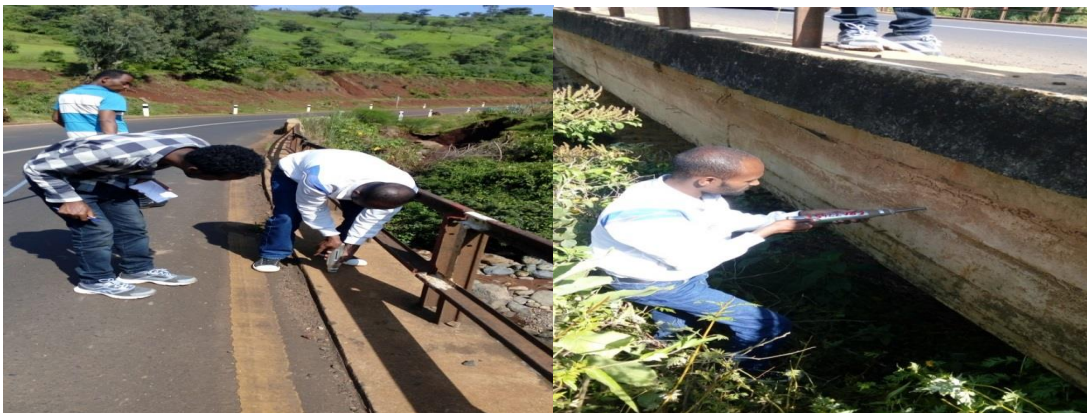
Figure 3.3 Taking Rebound hammer readings on Oda Bridge
