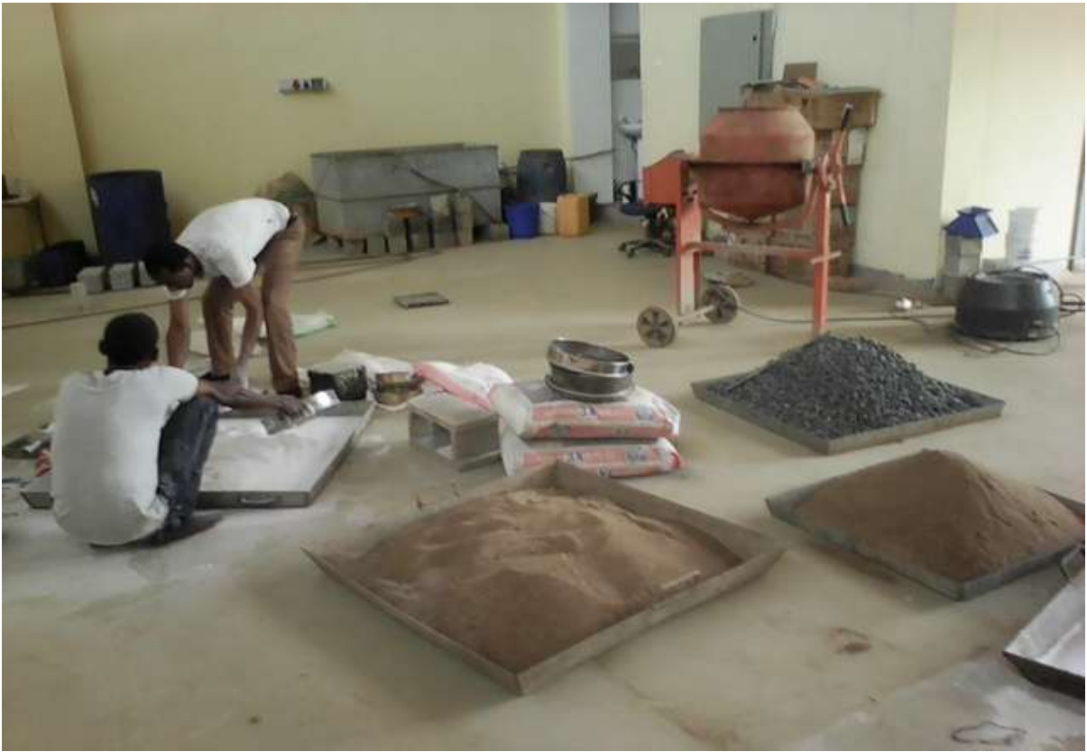
Photo 14: Over all Concrete making materials ready for mix.
