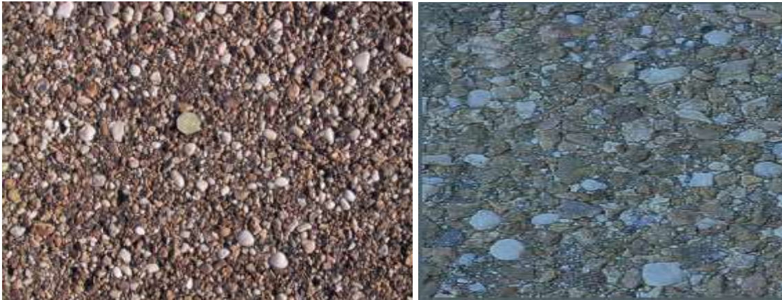
Figure 1: Matrix of Otta seal
