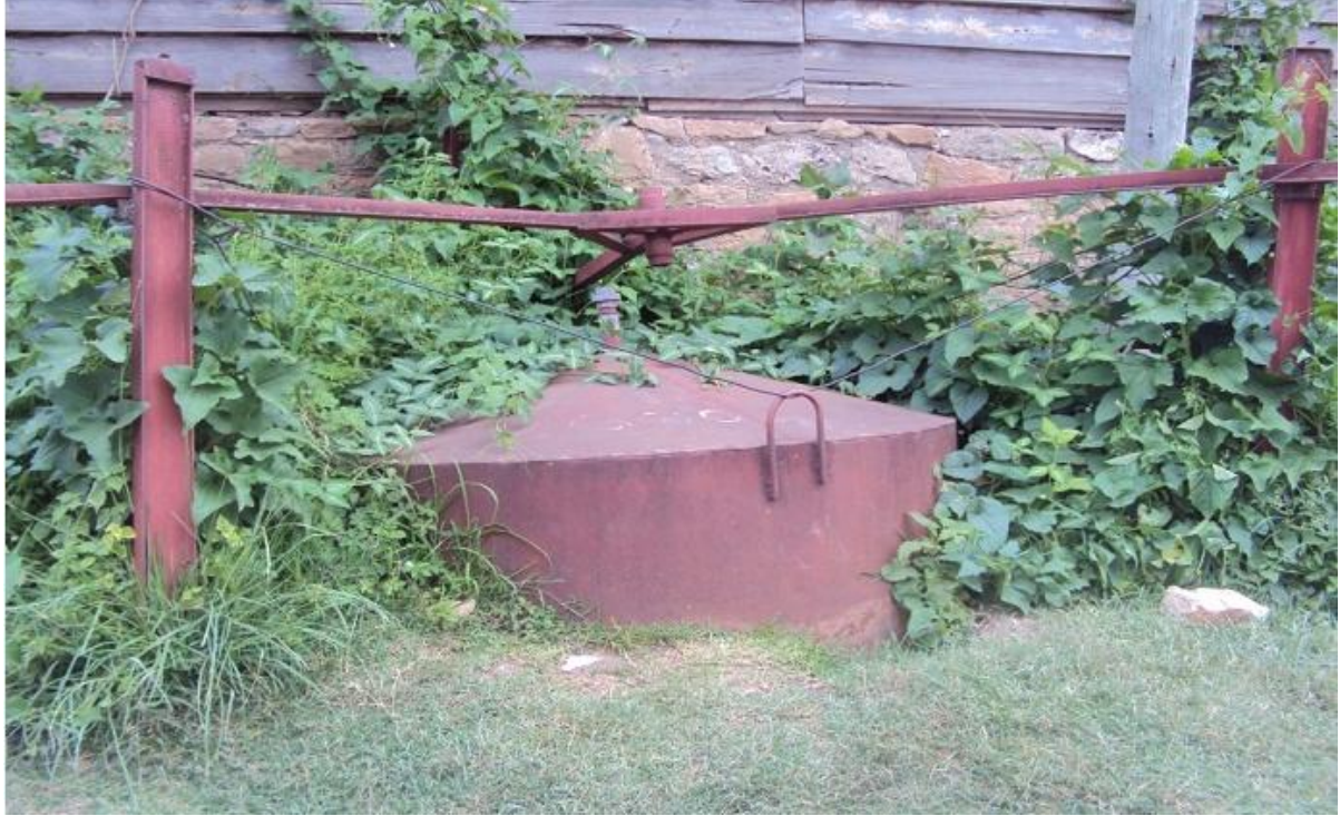
Figure 2: The first biogas plant installed in Ambo University (source; Meaza Ketsela Gebretsadik, 2012).
