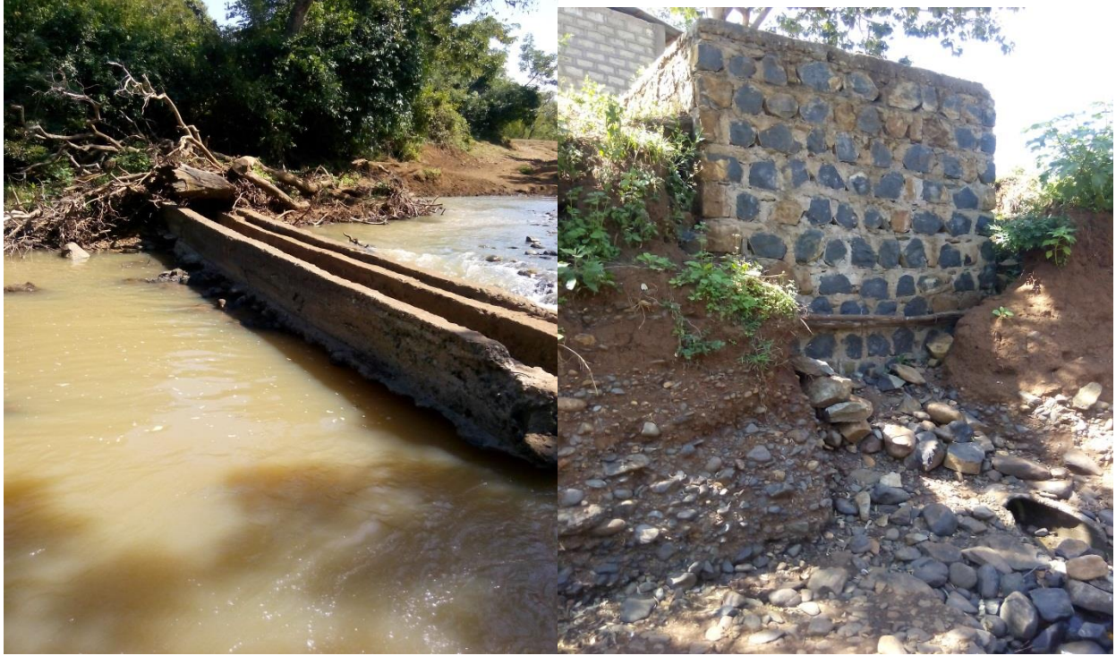
Figure1.5: Delivery channel, collection chamber and pump house.
