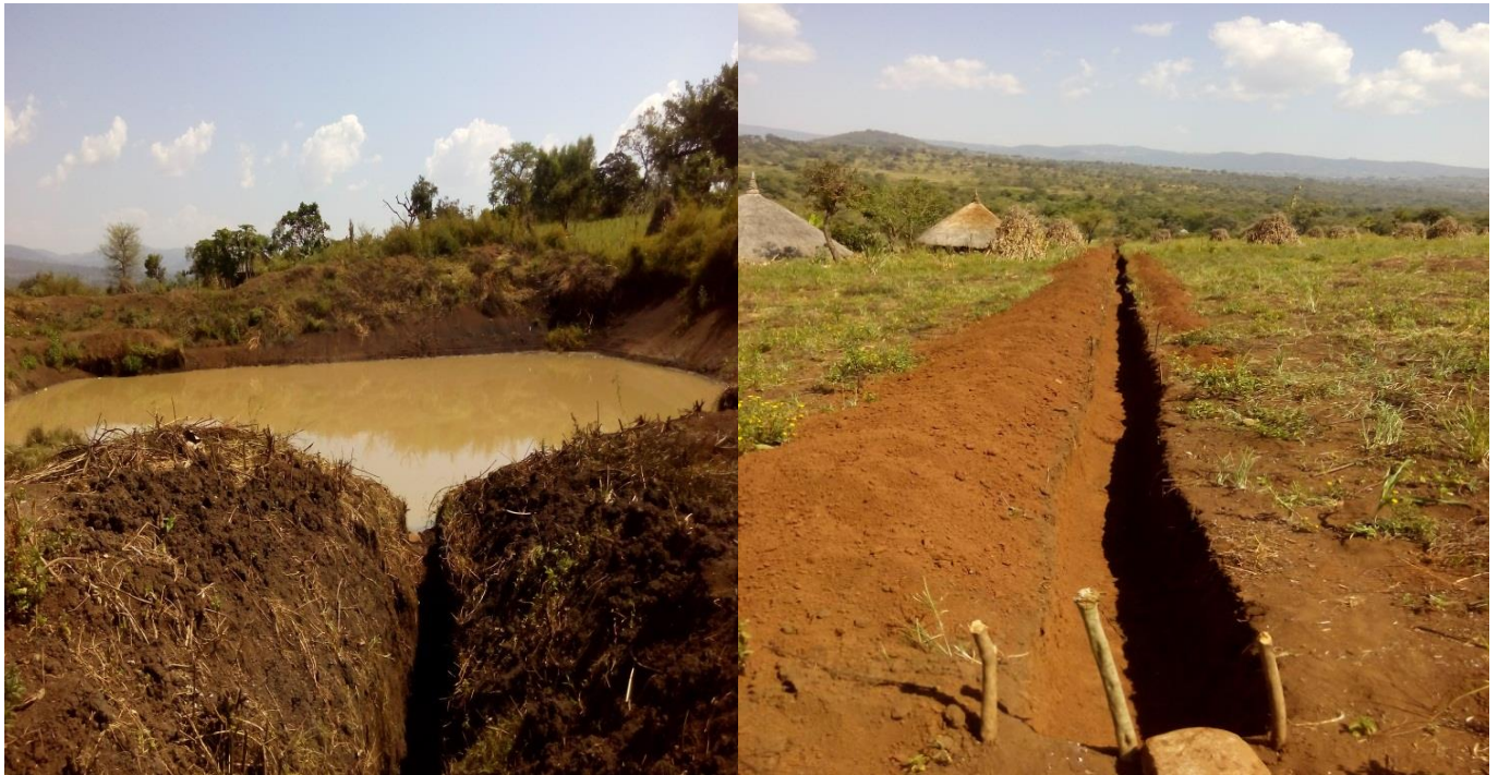
Figure1.8: Pond for water storage and delivery canal to agricultural lands of farmers.
