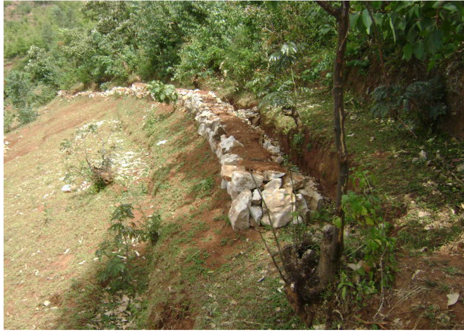
Fig. 8: Stone faced soil bunds on hill-side farm lands
